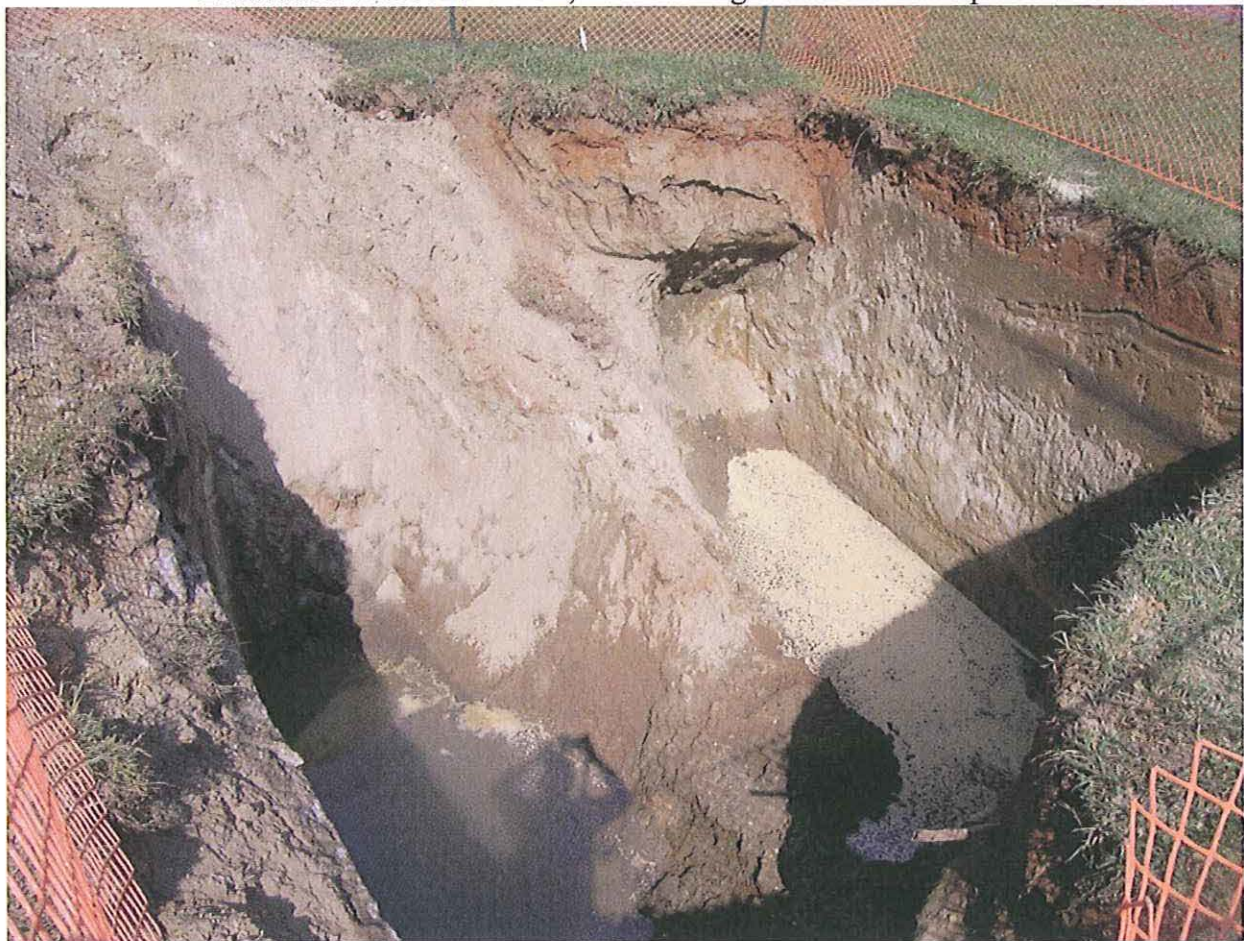
Completed remediation at 1123
