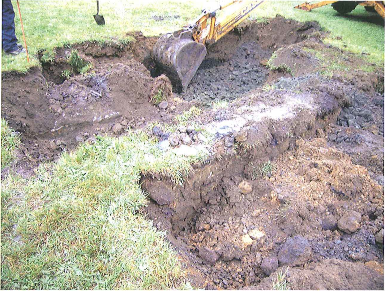
Test Pit at 537 looking for potential UHOT
