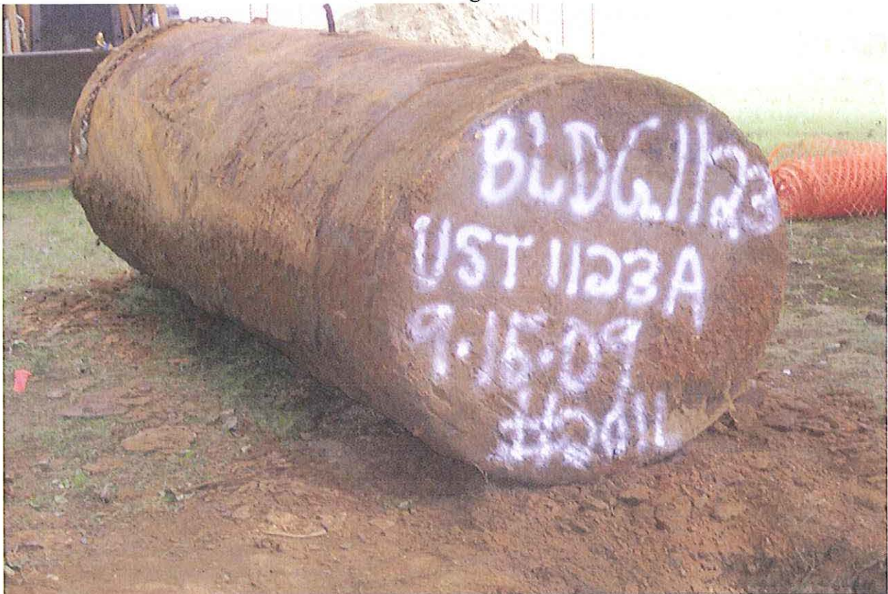
UHOT removed from excavation
