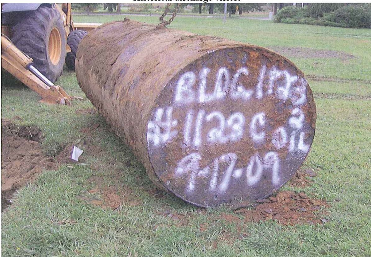
Second UHOT removed from Bldg. 1123
