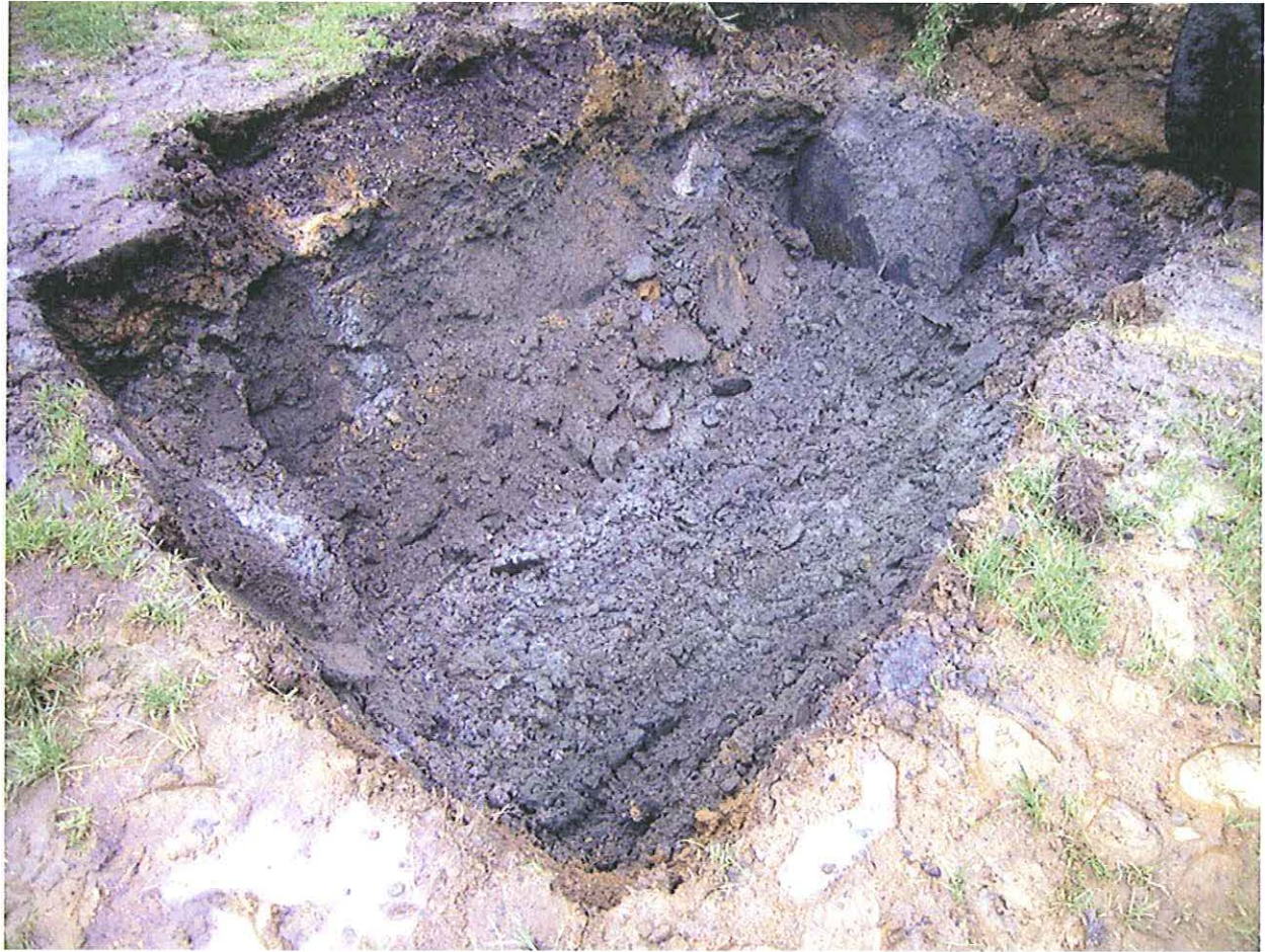
UHOT excavation after removal behind 542
