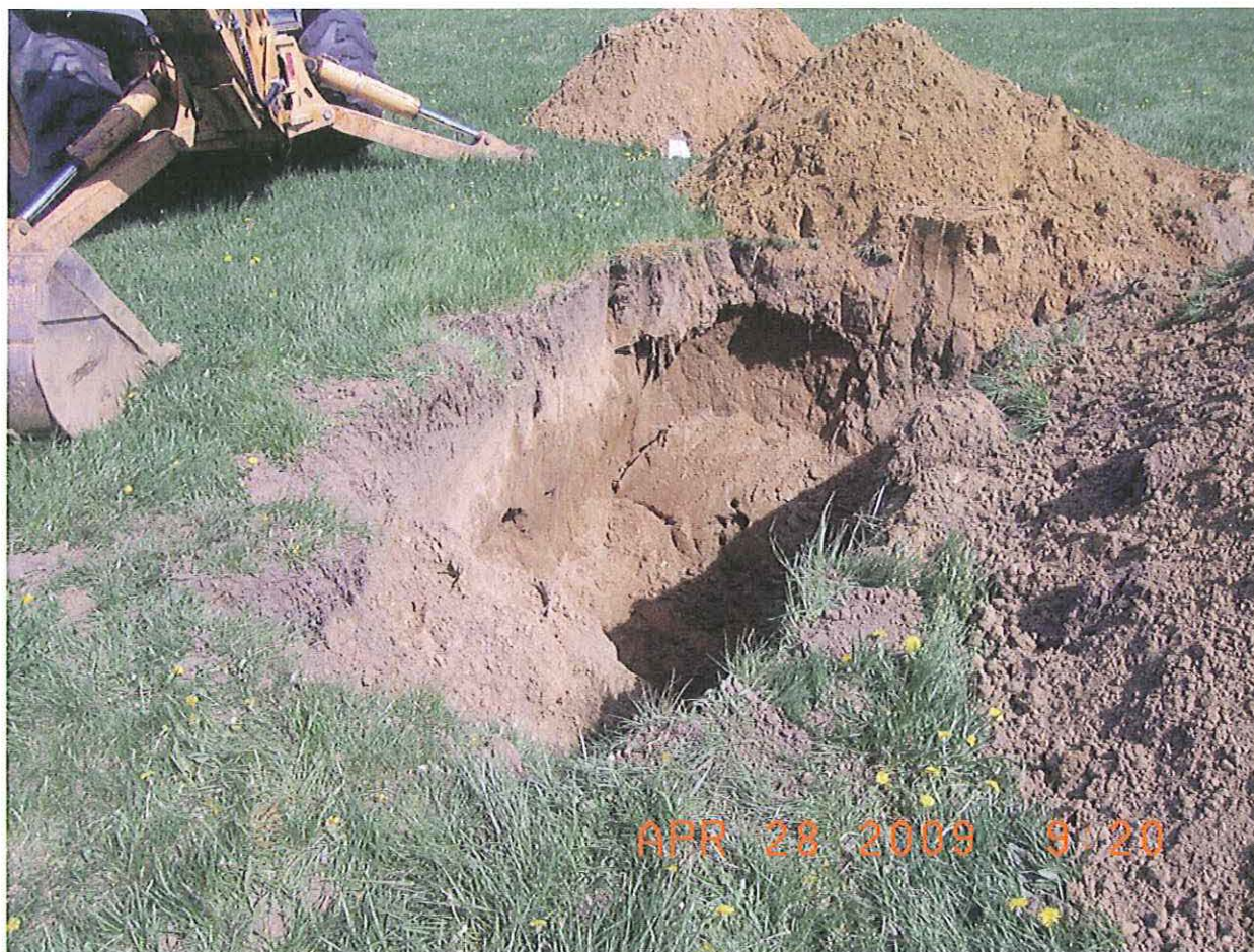
Clean excavation after removal of UHOT
