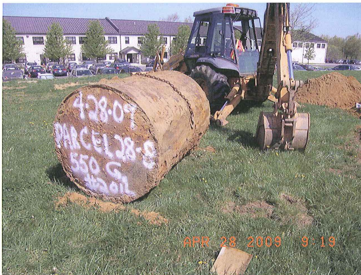
Tank removed from excavation, no visible holes present
