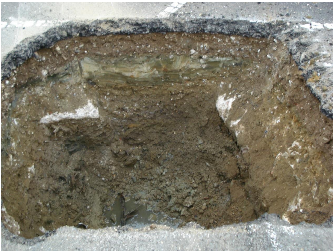
Photograph 9. Parcel 57, excavation completed, view north, 28 July 2016.
