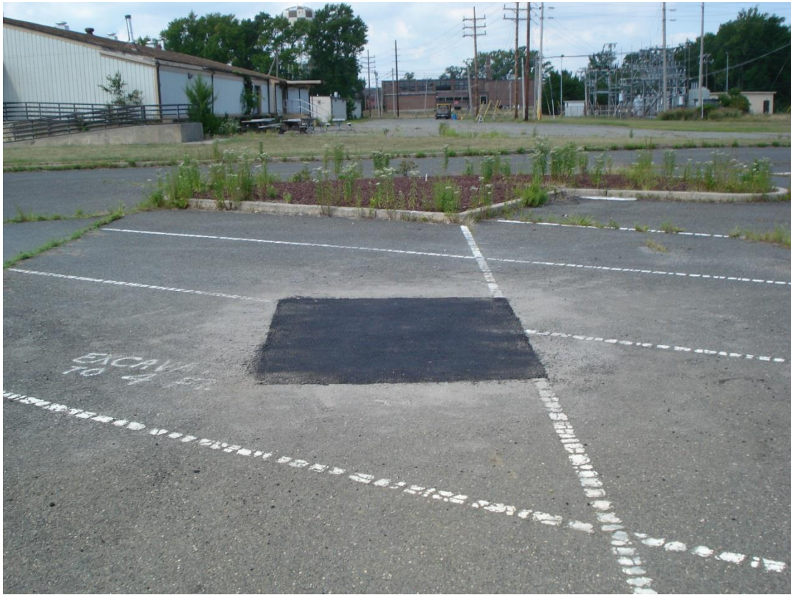
Photograph 13 – Parcel 57, excavation with asphalt patch, view west, 26 August 2016.
