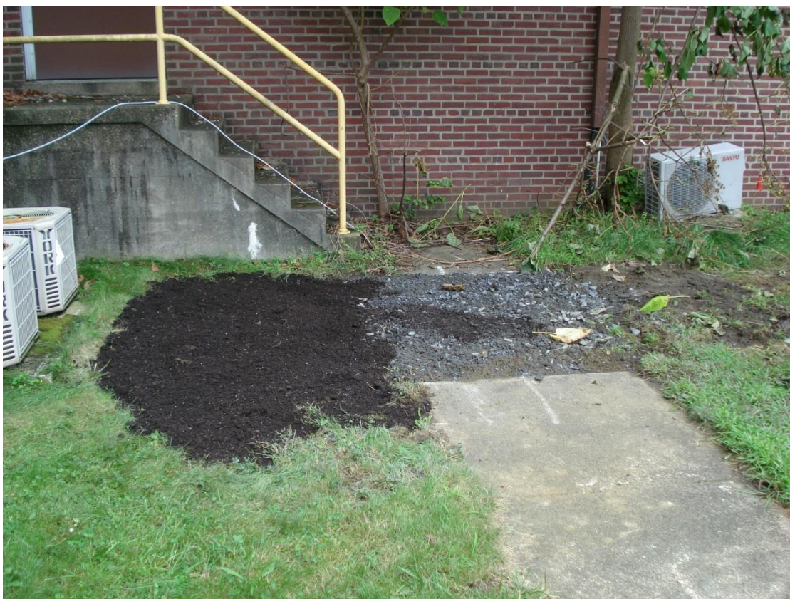
Photograph 4. Parcel 49, backfilled excavation, view west, 01 August 2016.
