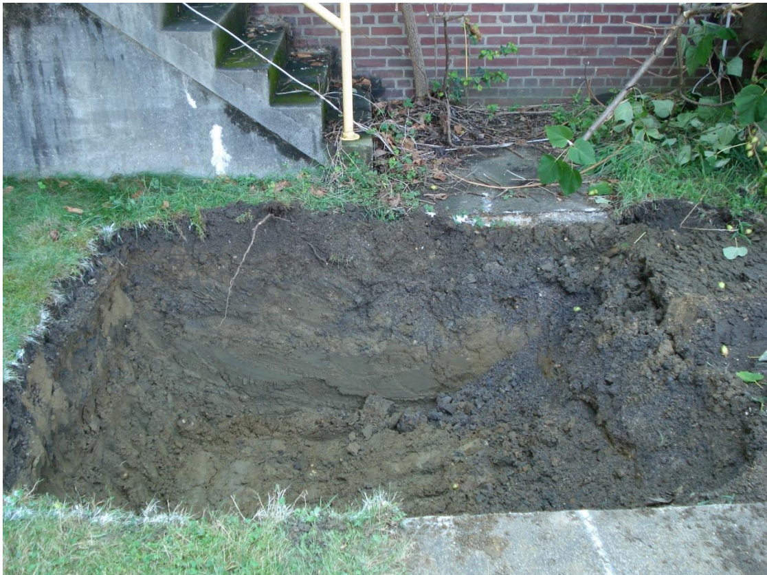
Photograph 2. Parcel 49, west wall of excavation, view west, 29 July 2016.
