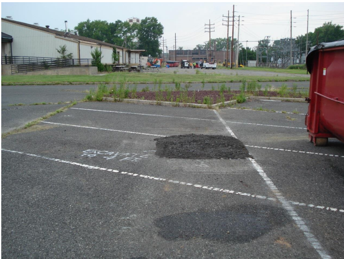
Photograph 12. Parcel 57, backfilled excavation, view west, 28 July 2016.
