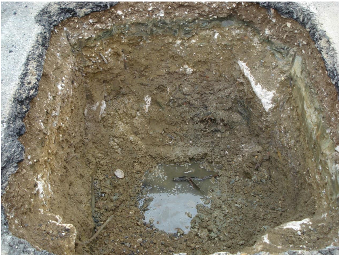
Photograph 11. Parcel 57, bottom of excavation with water seeping in, 28 July 2016.
