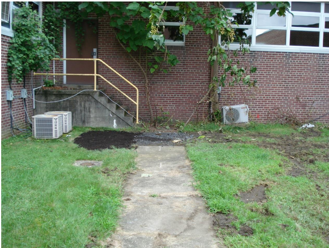
Photograph 5. Parcel 49, backfilled excavation and adjacent area, view west, 01 August 2016.
