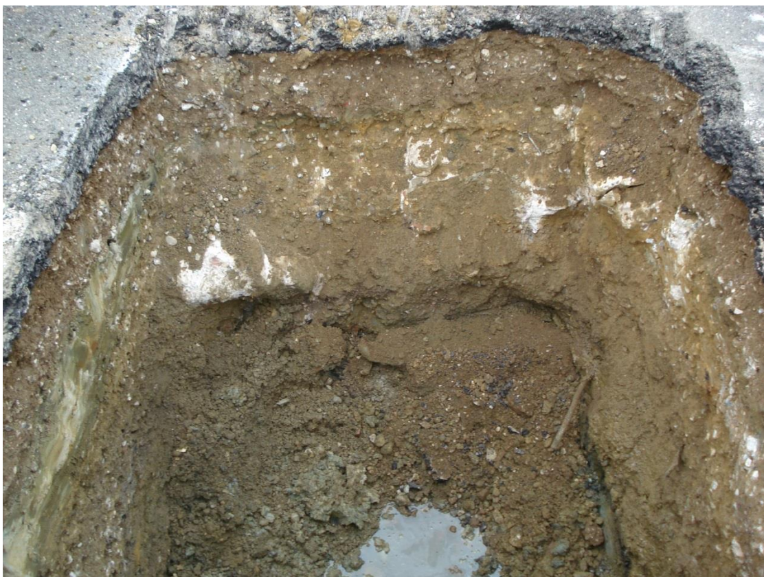
Photograph 10. Parcel 57, east wall of excavation, view east, 28 July 2016.
