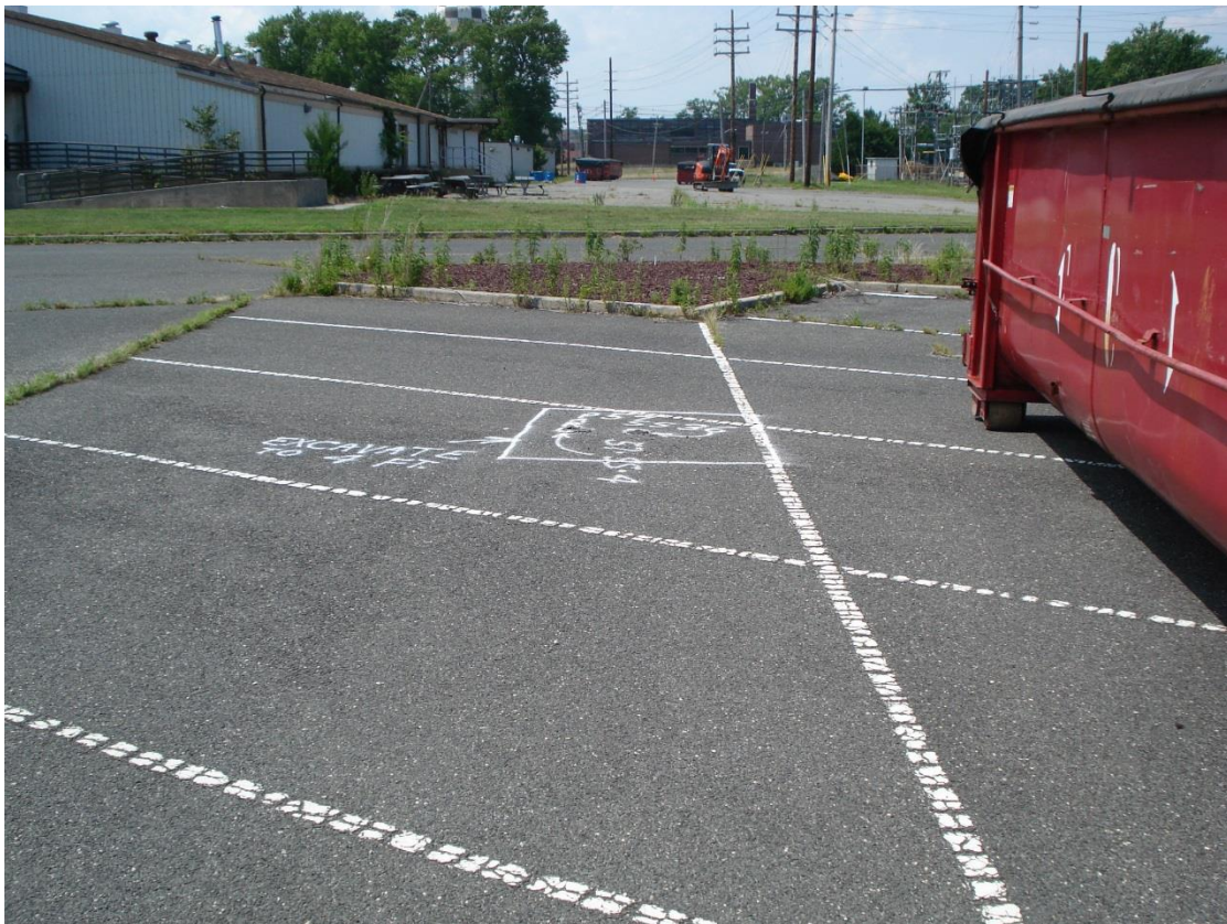
Photograph 7. Parcel 57, marked excavation area, view west, 28 July 2016.
