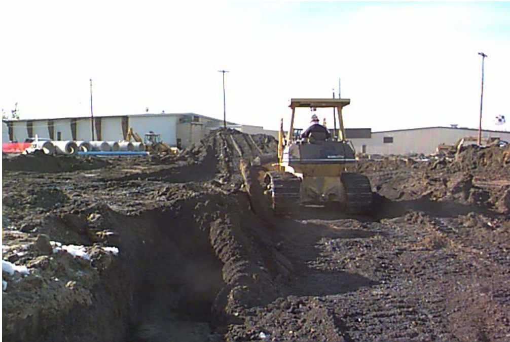
Jan 15, soil excavation from the fuel distribution/railroad track area. The contaminated material was excavated and transported to the ID-27 soil pile staging area.
