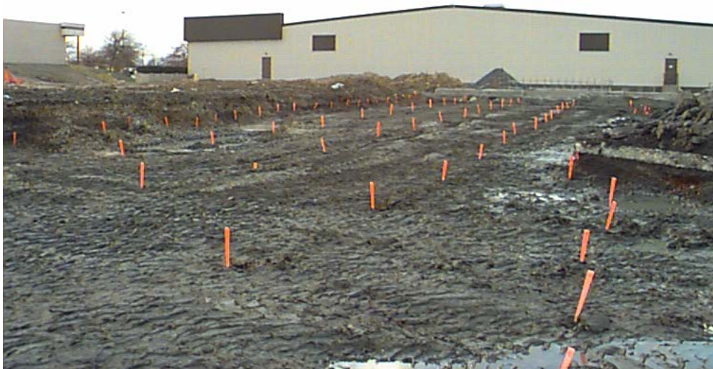
West excavation area (railroad track area)
