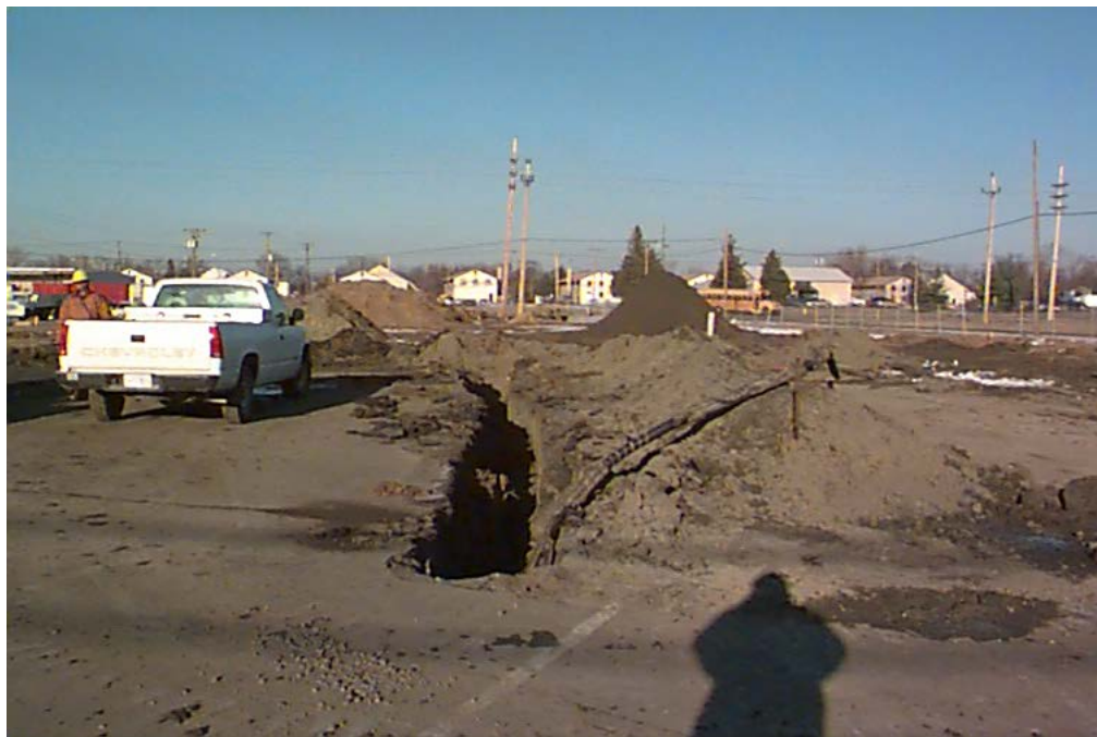
Jan 14, gas pipe excavation from the fuel distribution/railroad track area facing north. This pipe led us to the most contaminated area (the rail-car off-loading area) which is believed to be the source area for the fuel contamination.
