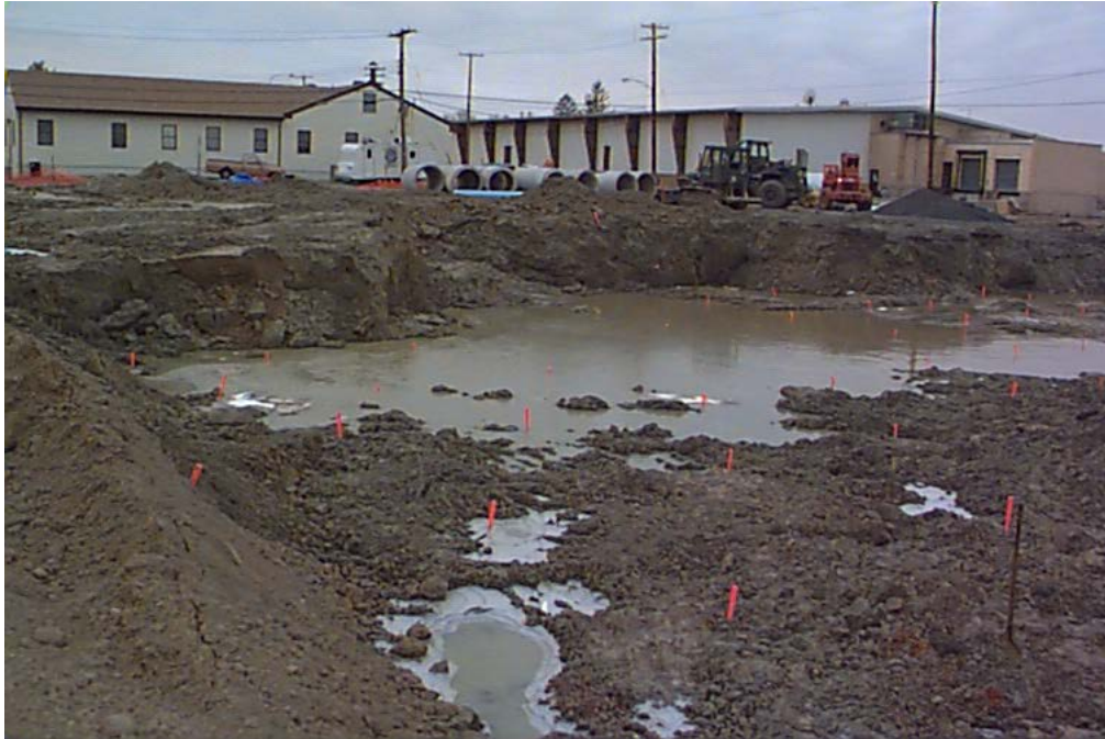
Central excavation area (fuel distribution/railroad track area) sample results show a clean excavation and the area is being backfilled._
