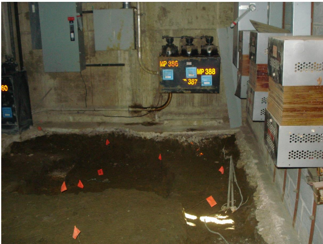
Photograph 5. Building 1209, PCB soil sample locations, view south, 2 August 2016.
