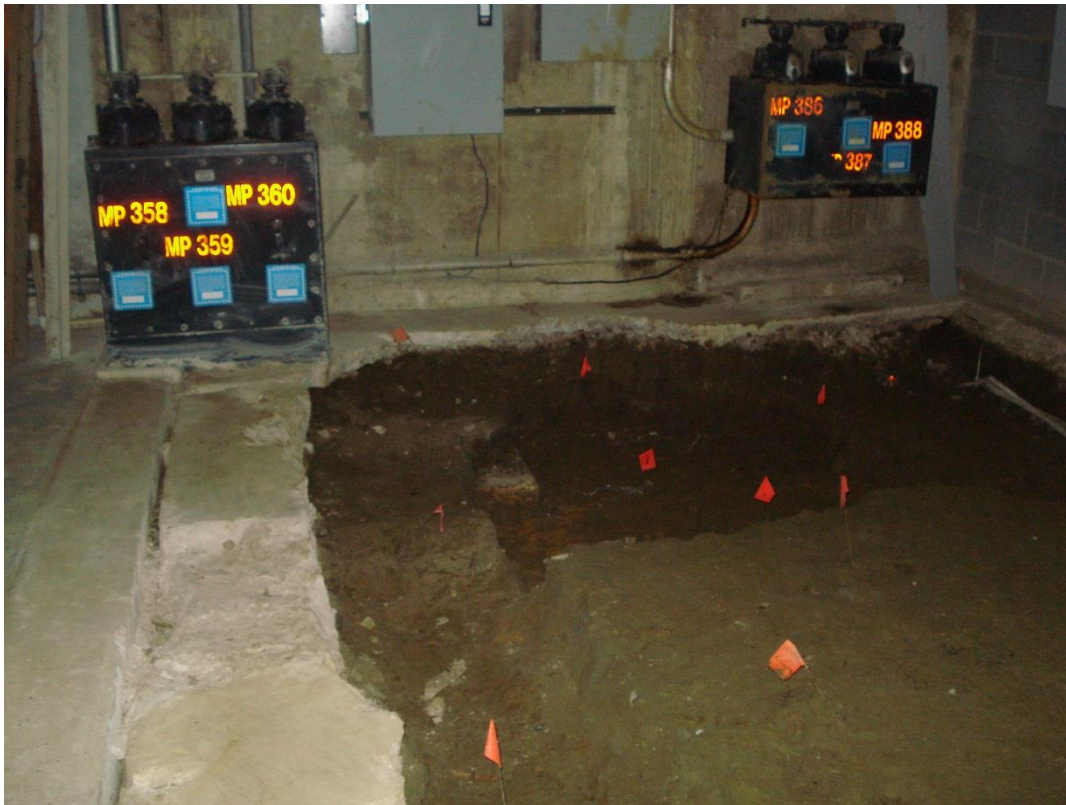
Photograph 4. Building 1209, PCB soil and concrete sample locations, view south, 2 August 2016.
