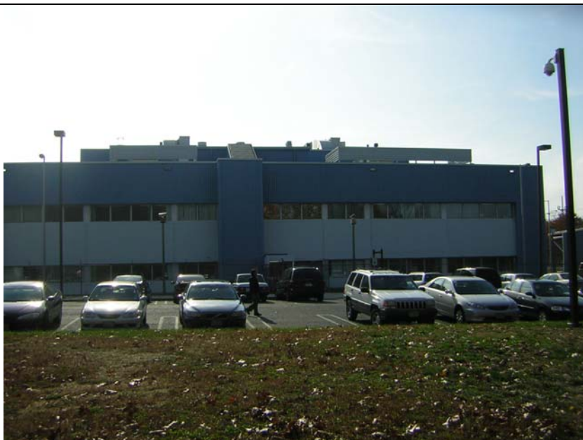
Building 2707, Main (North) Elevation S View
