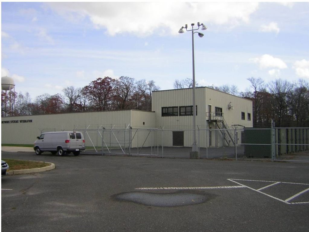
Figure 4-4: South end of EWL Showing 2-Story Rectangular Projecting Bay, Looking Northeast
