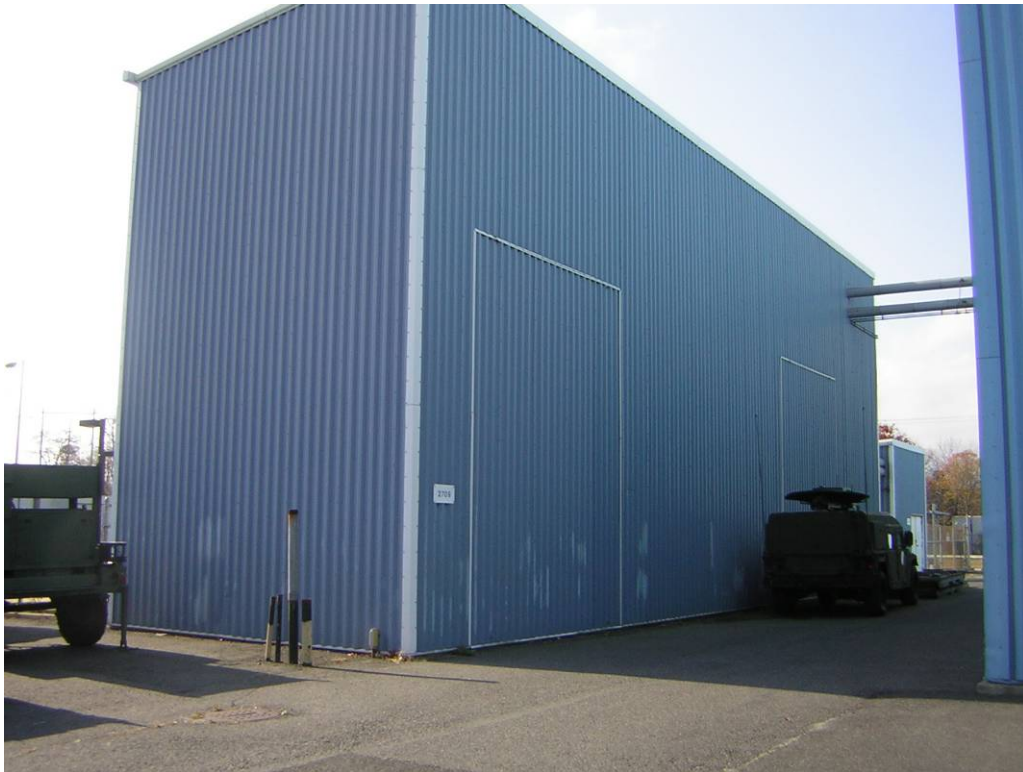
Figure 4-11: Building 2709, North and East Elevations, Looking Southwest
