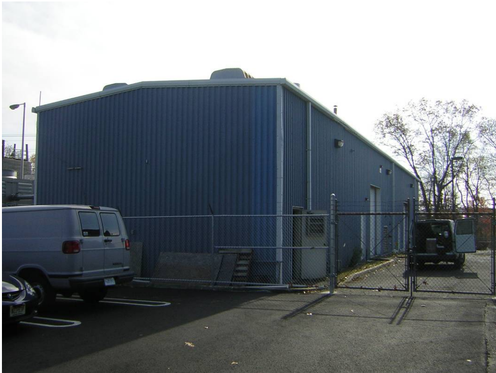
Figure 4-10: Building 2708, North and West Elevations, Looking Southeast
