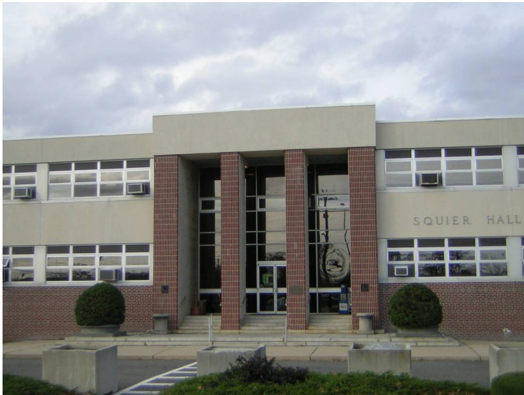
Figure 4-16: Squier Hall (Building 283), Detail of Front or South Elevation, Looking Northwest
