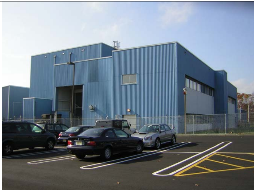
Building 2707, East Elevation SW View
