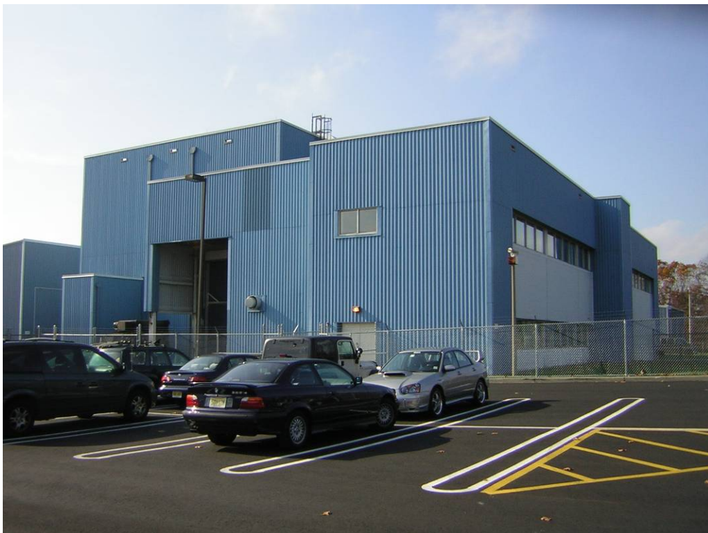
Figure 4-8: Building 2707, East Elevation, Looking Southwest
