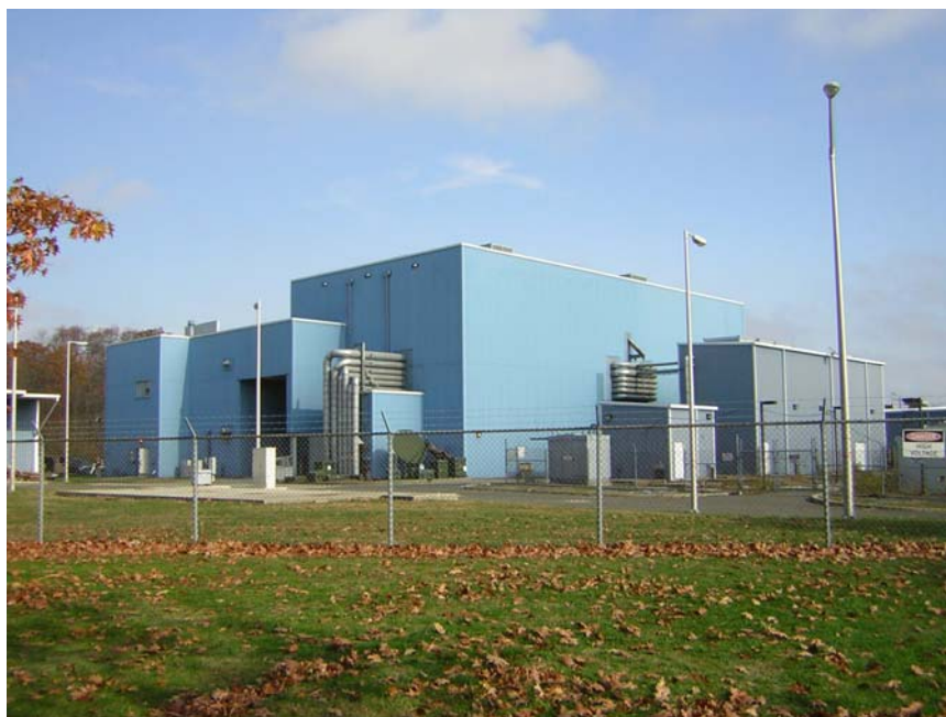
Building 2707, South and West Elevations, NW View
