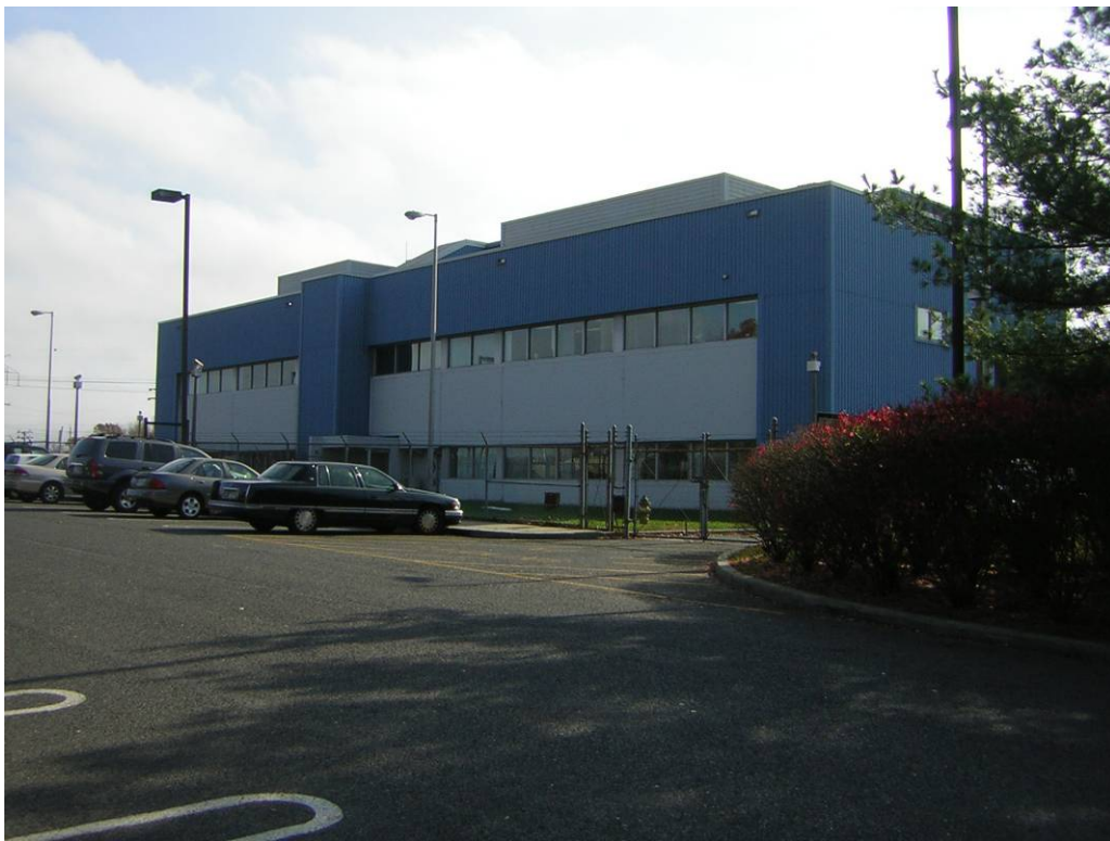
Figure 4-6: Building 2707, North Elevation, Looking Southeast.
