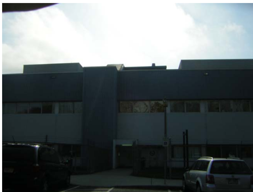
Building 2707, Main Entrance on North Elevation, SE View
