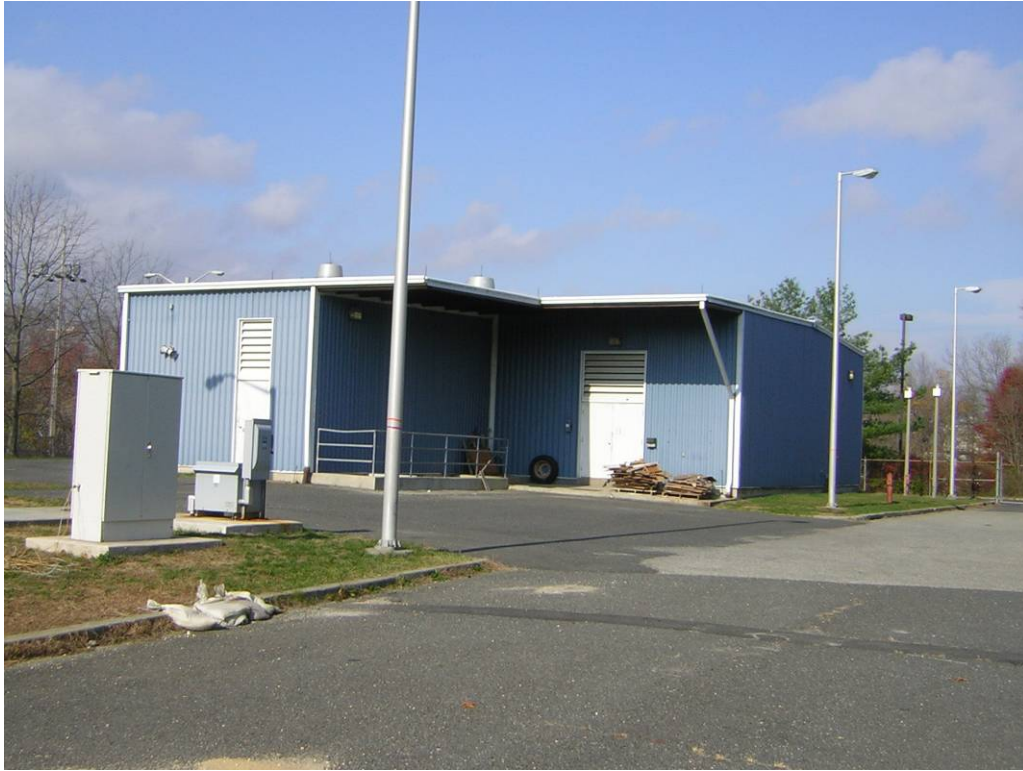
Figure 4-13: Building 2713, South and East Elevations, Looking Northwest
