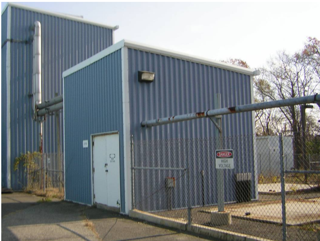
Figure 4-12: Building 2710, North and West Elevations, Looking Southeast
