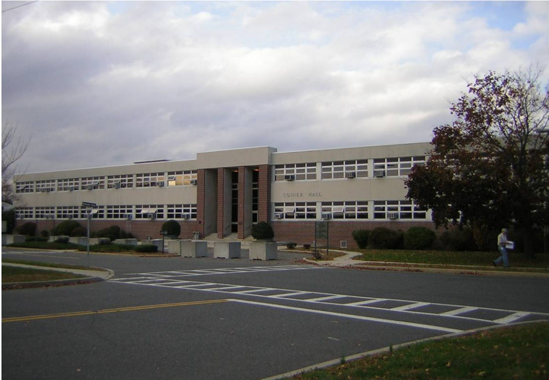
Figure 4-15: Squier Hall (Building 283), Front or South Elevation, Looking Northwest
