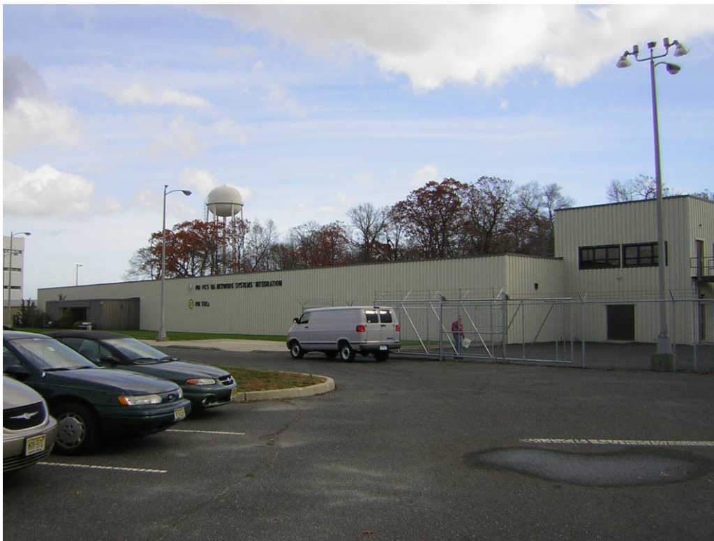
Figure 4-2: EWL (Building 2705), West Elevation, Looking Northeast
