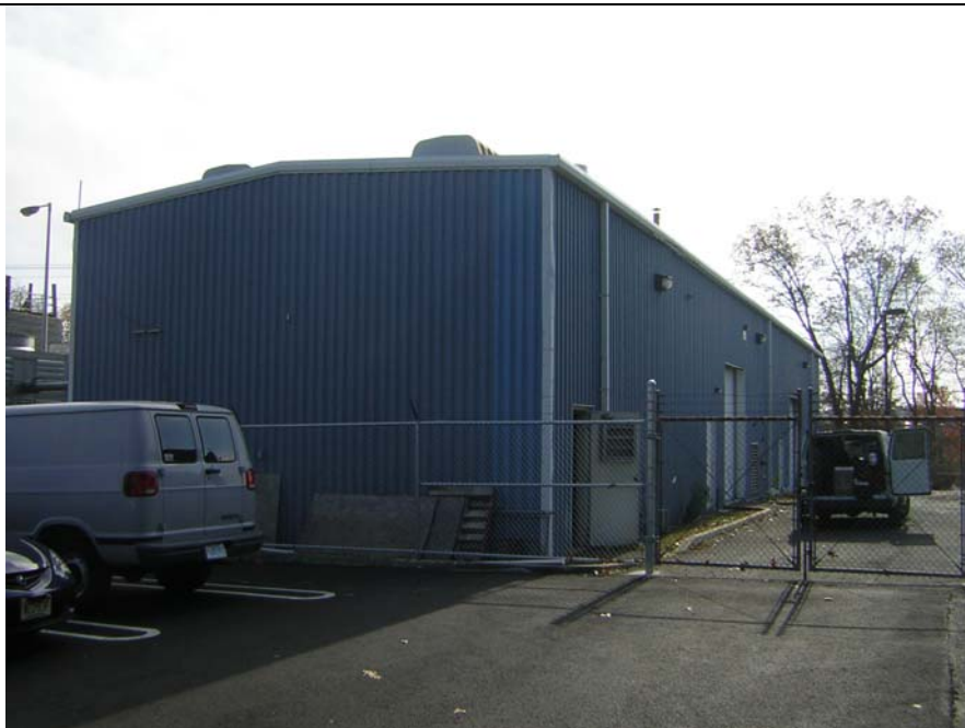
Building 2708, North and West Elevations S View
