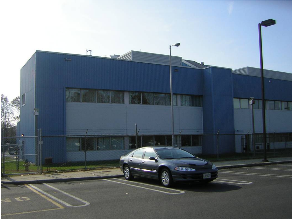
Figure 4-7: Building 2707, North Elevation Detail, Looking South.
