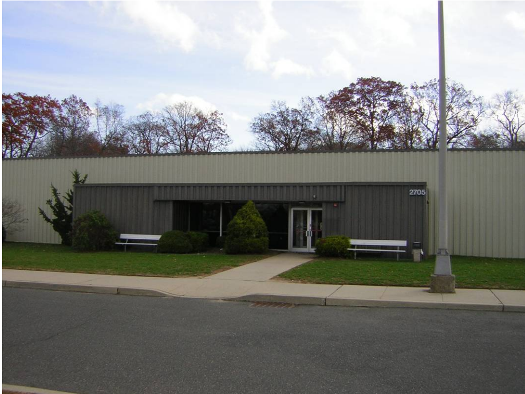
Figure 4-3: Main Entrance to EWL, Looking East
