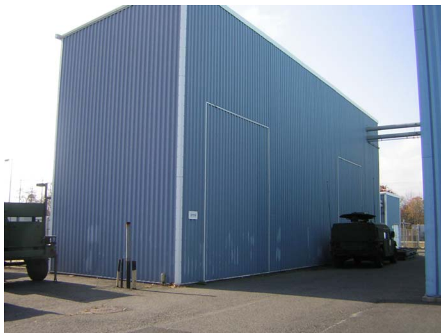
Building 2709, North and East Elevations, SW View
