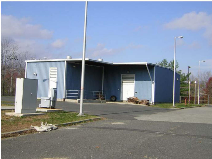
Building 2713, South and East Elevations, NW View
