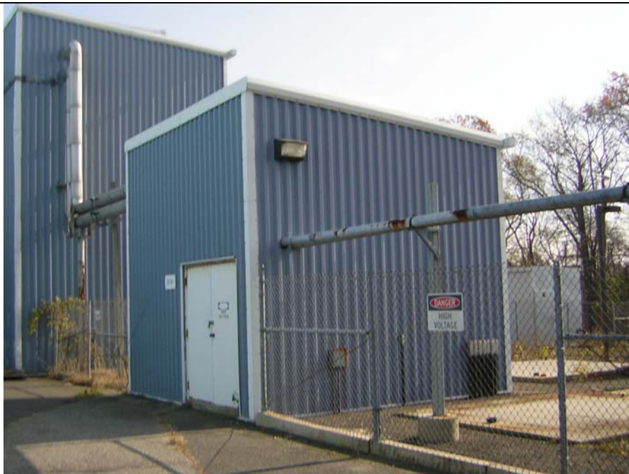
Building 2710, North and West Elevations SE View
