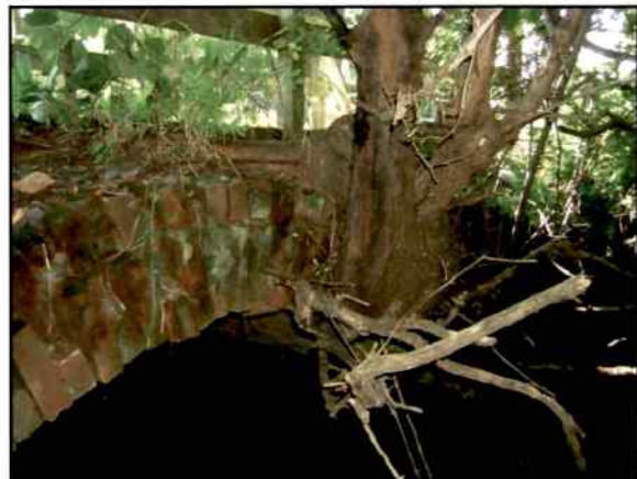
Figure 4-13. Site 28MO385, Brick Culvert, View South Showing Tree Growth from Facing of Arched Superstructure
