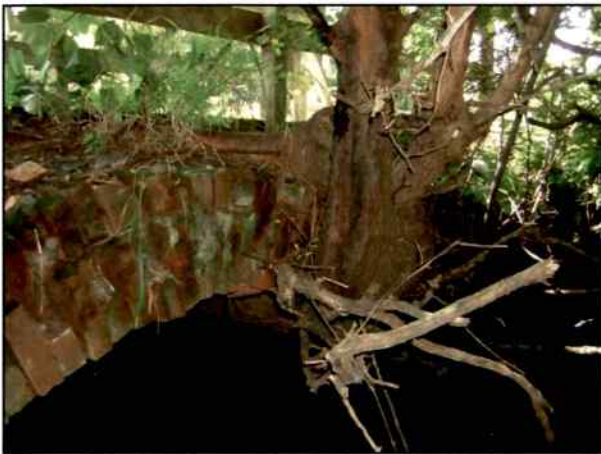
Figure D. Brick Culvert, View South Showing Tree Growth from Facing of Arched Superstructure.
