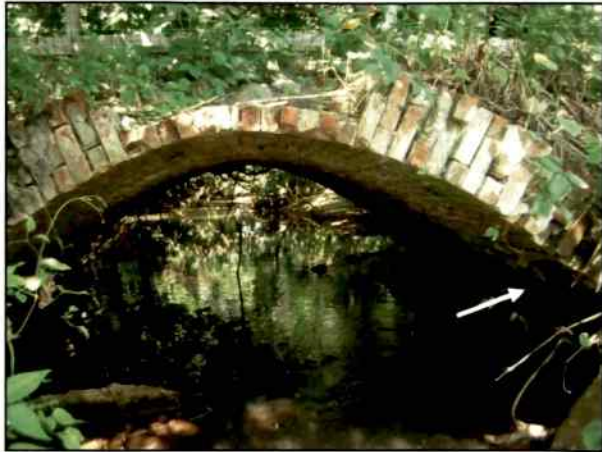
Figure D. Brick Culvert, View South Showing Tree Growth from Facing of Arched Superstructure.
