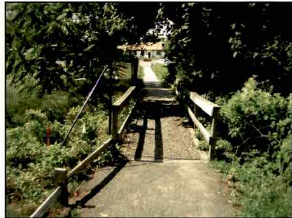
Figure 4-11. Site 28MO385, Modern Pedestrian Bridge over Brick Culvert, View West
