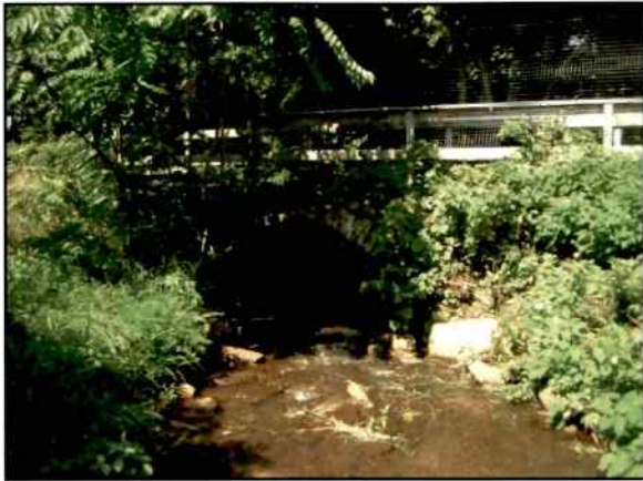
Figure 4-10. Site 28MO385, Brick Culvert, View North from Husky Brook
