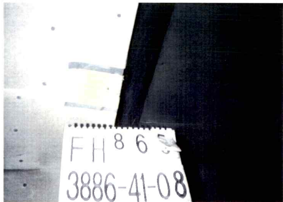
BOILER ROOM: (SAMPLE FH865 AND FH866) TRANSITE PANELS TESTED POSITIVE.
