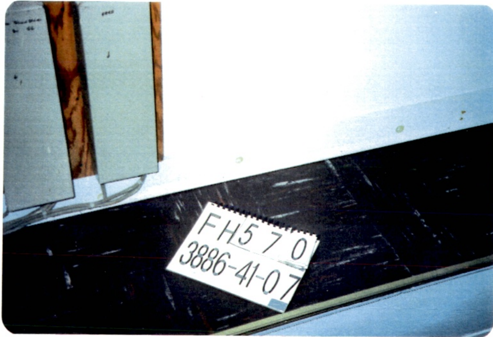
Bldg. 9015 - EW RSTA: 9 x 9" brown floor tiles FH570 tested positive.
