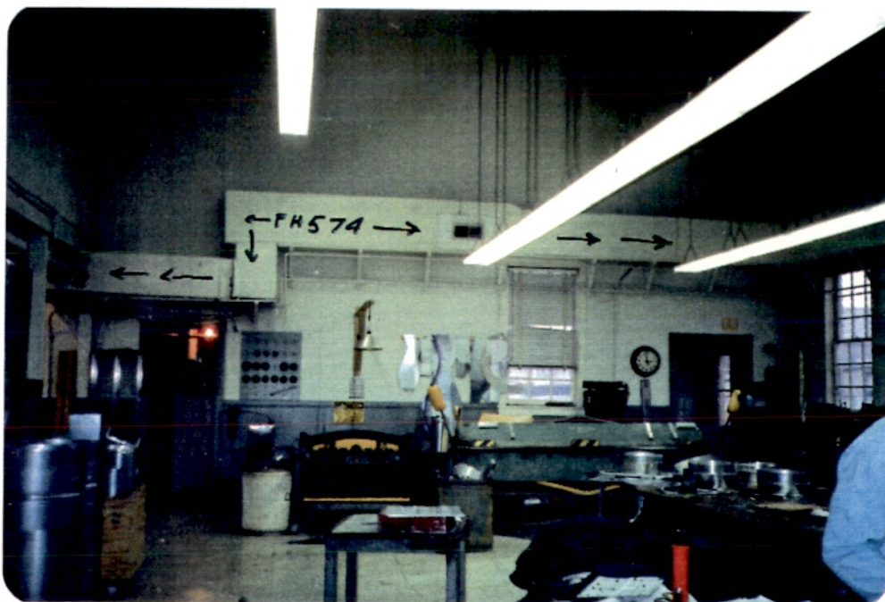
Bldg. 9023 - Metal Shop: Duct insulation sample FH574 tested positive; also sample FH572, 12 x 12" tan floor tiles in shop area tested positive. Sample FH573, 12 x 12" tan floor tiles upstairs offices (FH572 and FH573 not shown).
