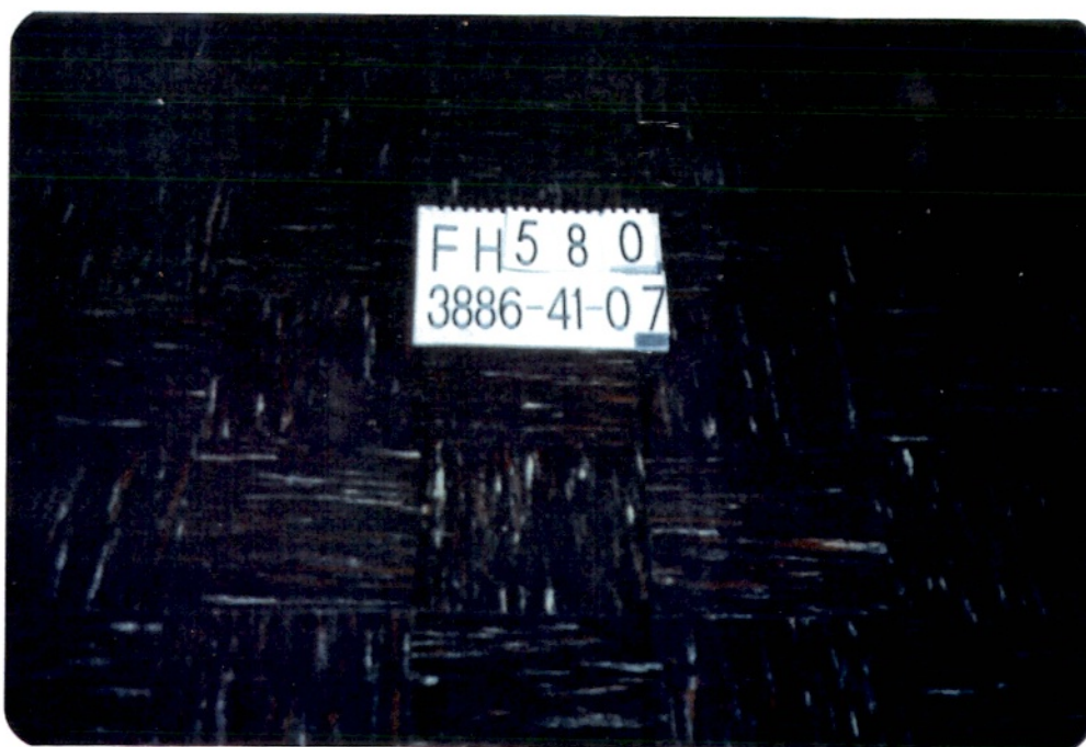
Bldg. 9009 - Serv-Air Garage/Shop: 9 x 9" floor tiles sample FH580 tested positive.
