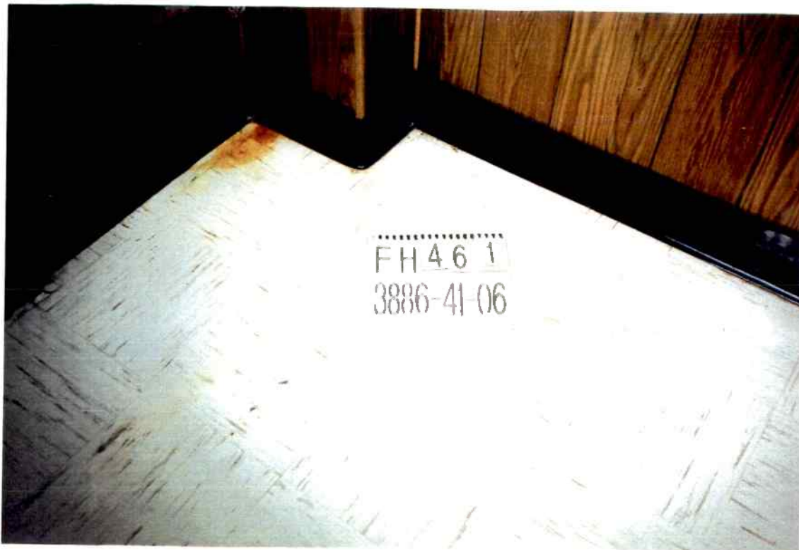
Bldg. 918: 12 x 12" tan floor tile with 9 x 9" brown floor tile below tested positive.
