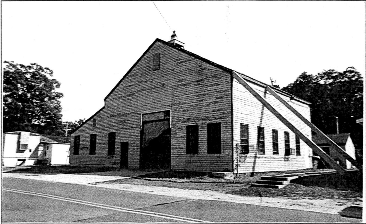
Figure 3.14 World War II-Era Buttressed Wooden Radar Building, 1996.
