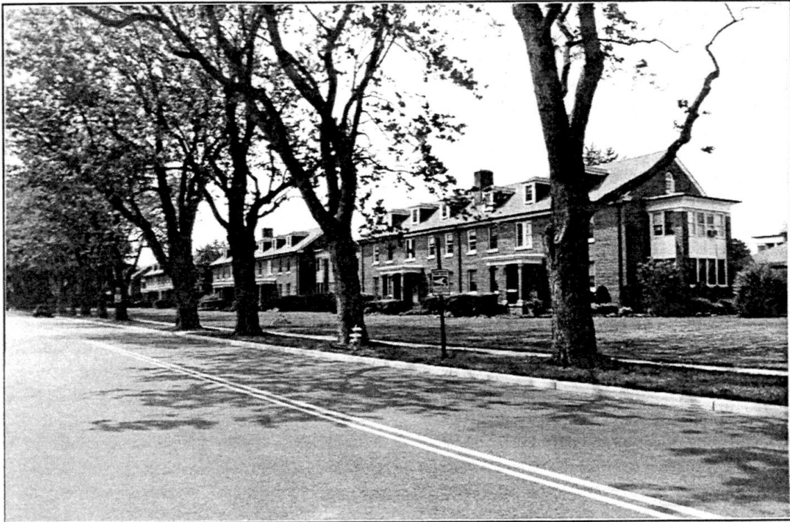
Figure 3.8 Duplex Officers Housing Within the Main Post National Register District.
