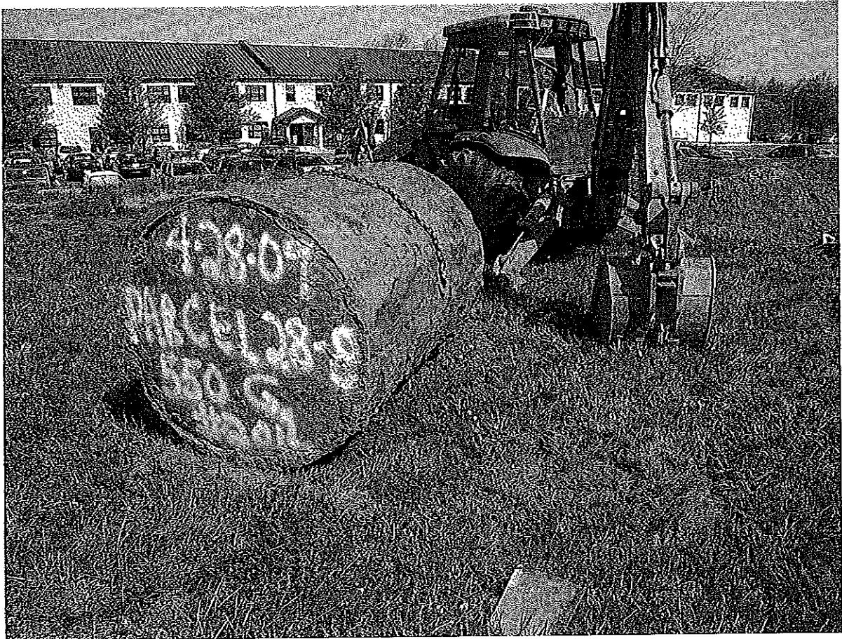
Tank removed from excavation, no visible holes present
