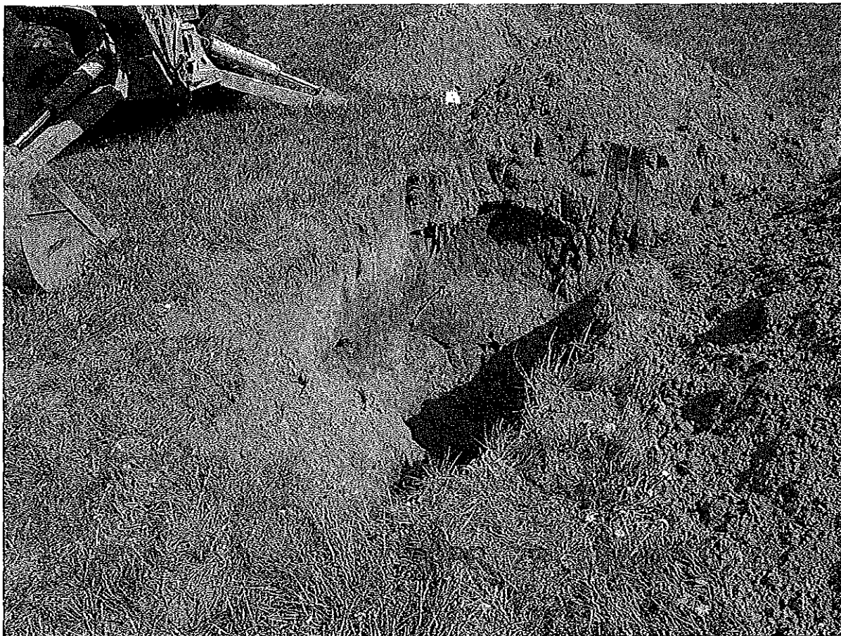
Clean excavation after removal of UHOT
