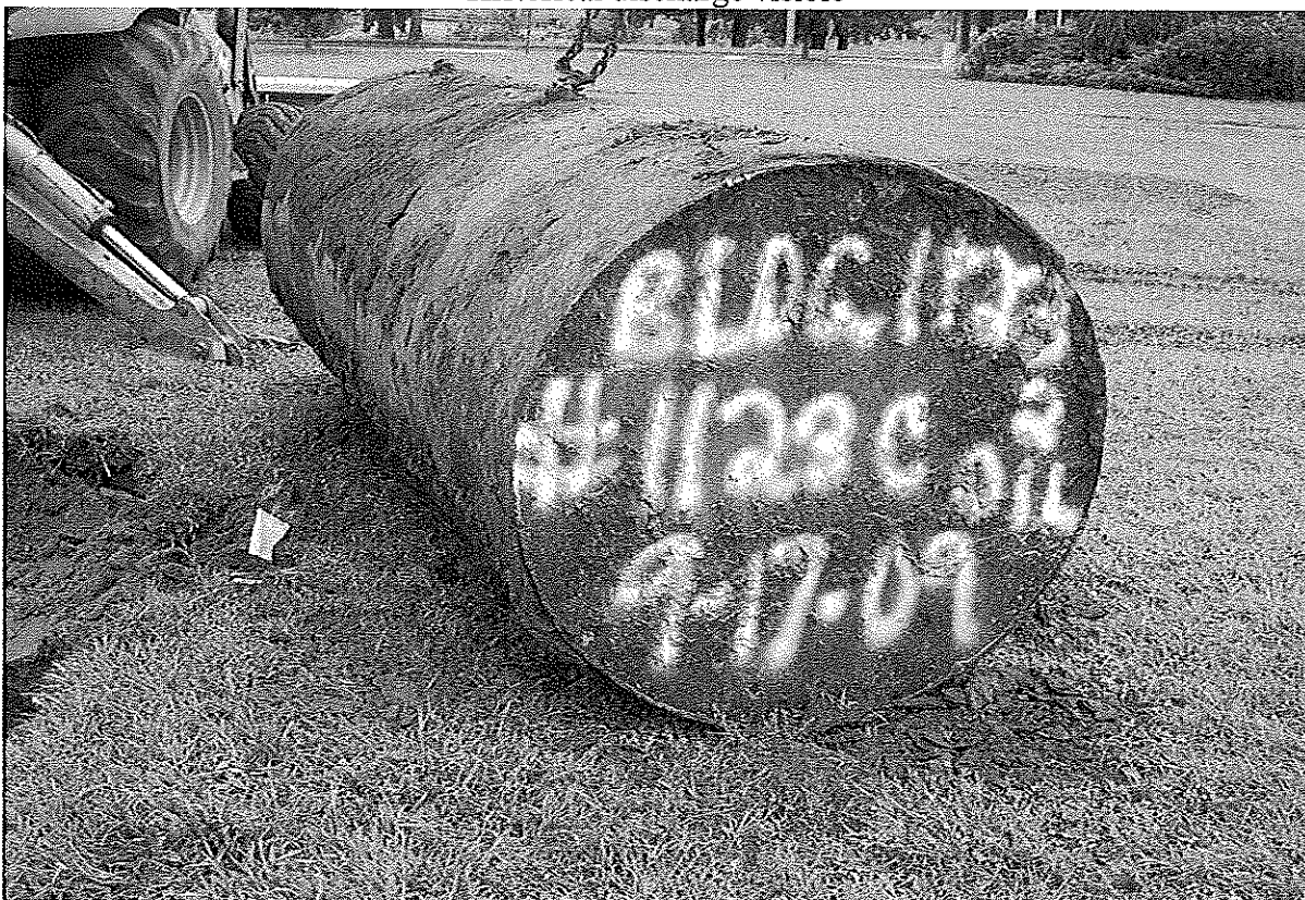
Second UHOT removed from Bldg. 1123
