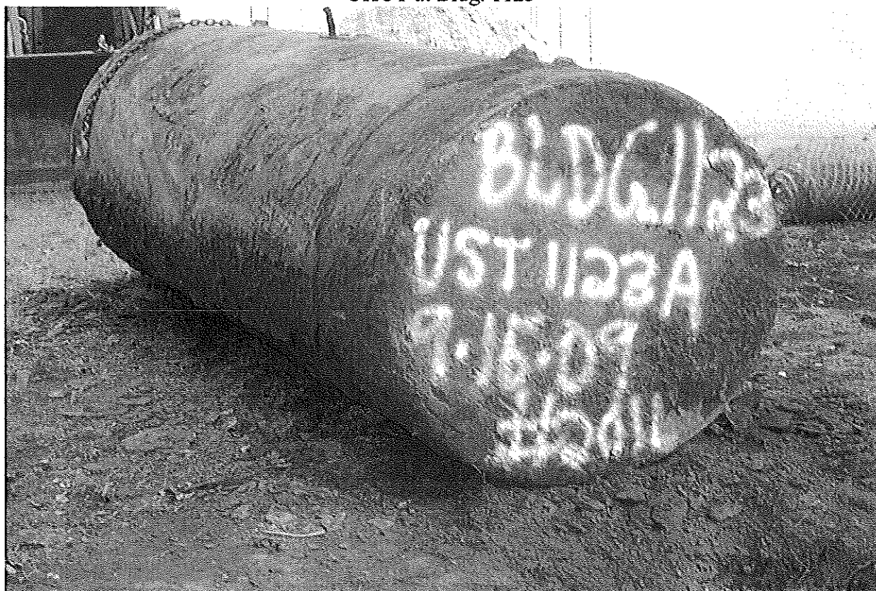
UHOT removed from excavation
