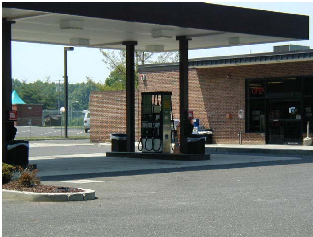
BUILDING 2567 AND GASOLINE PUMPS
