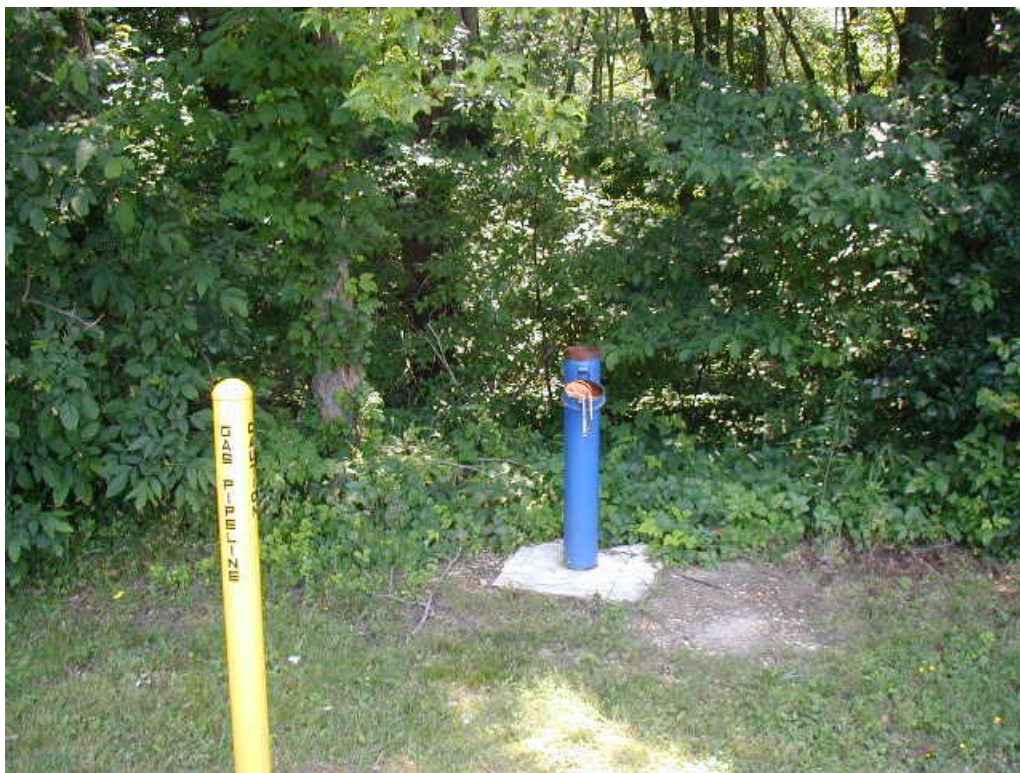
MONITORING WELL 2567-MW7
