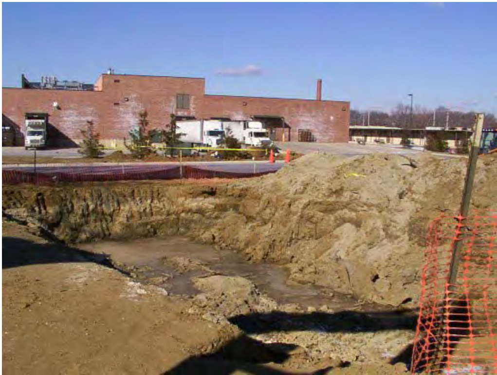
Photo #7: Looking North - Excavation in Grass Area
