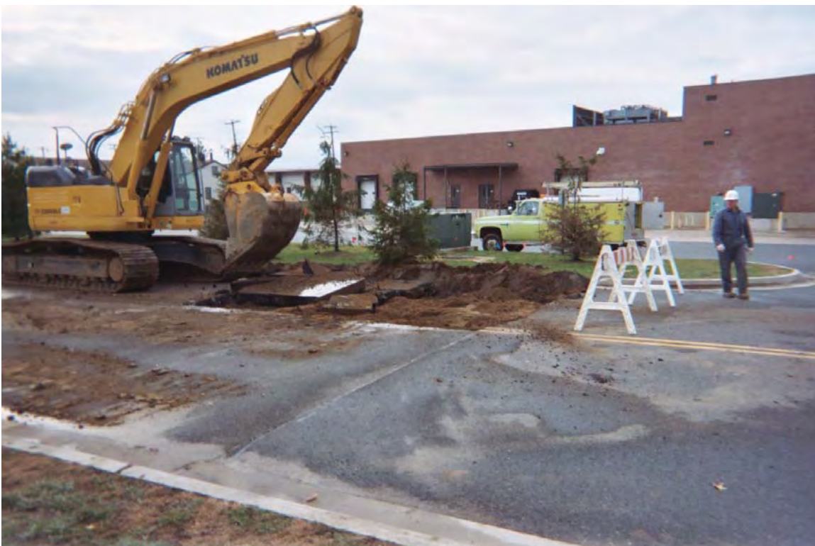
Photo #2: Looking West - Actively Excavating Murphy Drive
