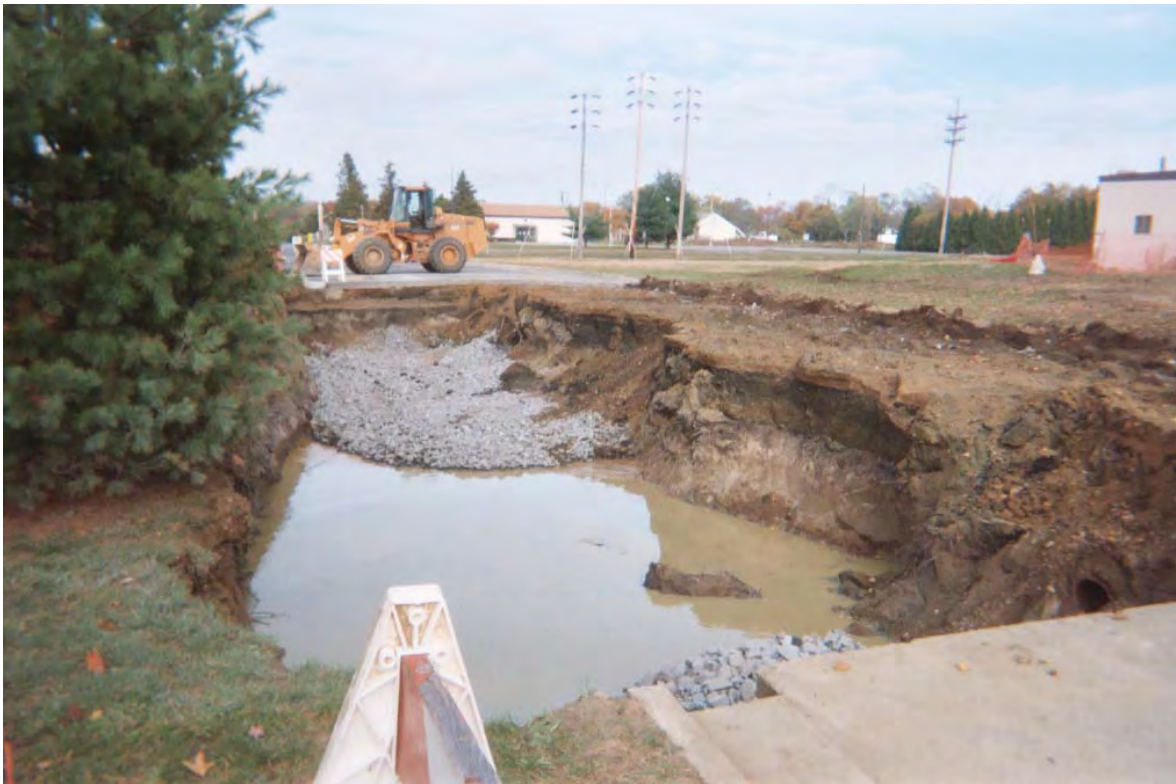
Photo #4: Looking Northeast - Actively Excavating Murphy Drive and Grass Island
