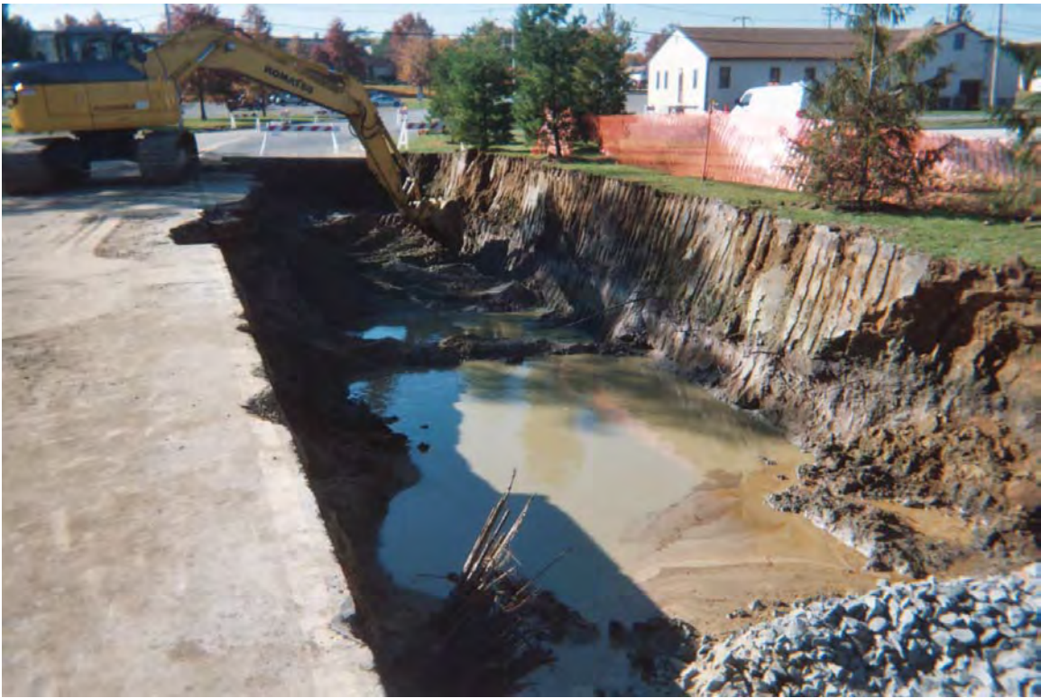
Photo #3: Looking Southwest - Actively Excavating Murphy Drive and Grass Island
