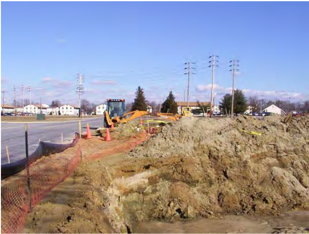
Photo #5: Looking East - Actively Excavating Grass Area Southeast side of Murphy Drive
