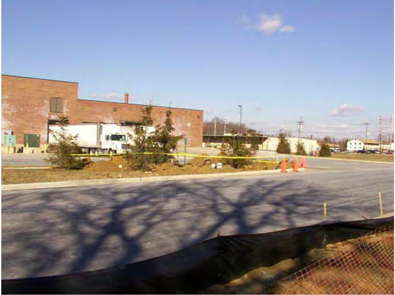
Photo #9: Looking North - Murphy Drive Restored
