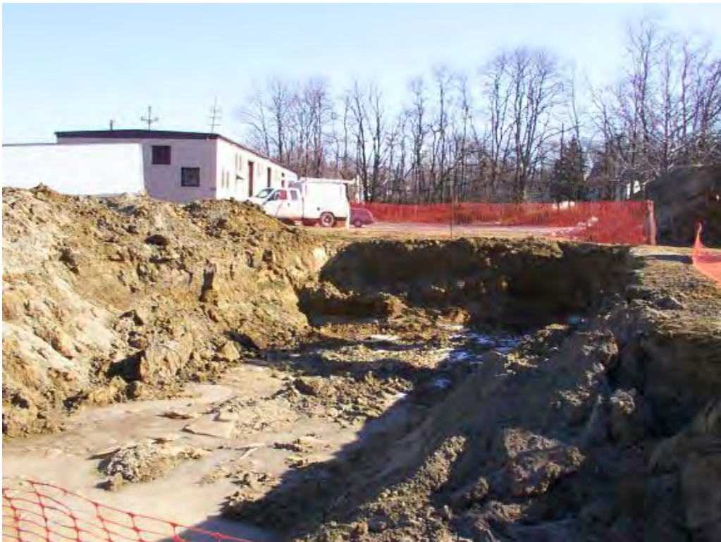
Photo #6: Looking Southeast - Excavation in Grass Area; Bldg. 886 in Background
