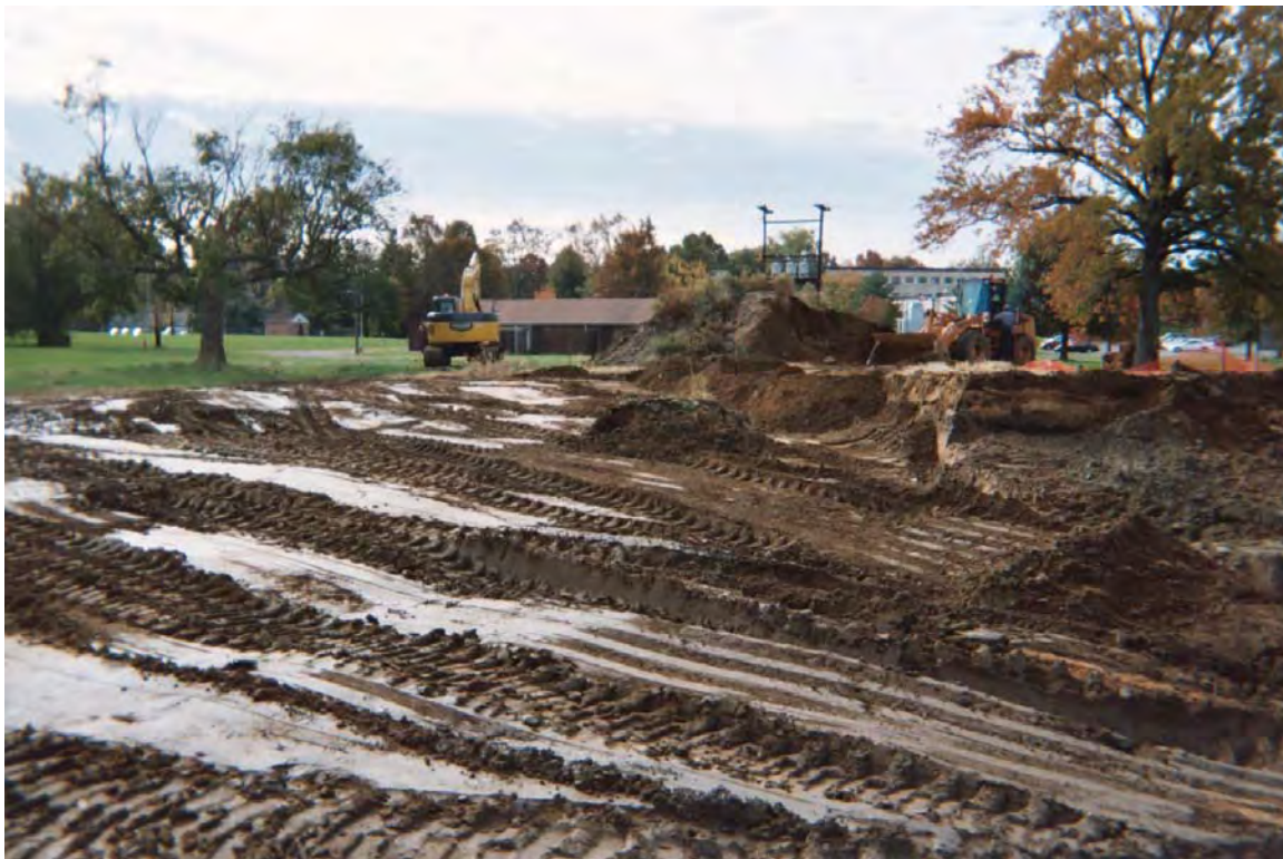
Photo #8: Looking South - Backfilling of Excavation
