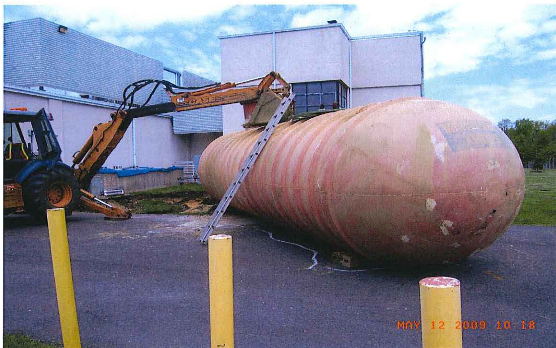
UST on ground ready for SSE inspection
