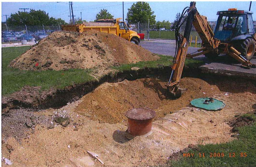
Exposing top of UST prior to removal
