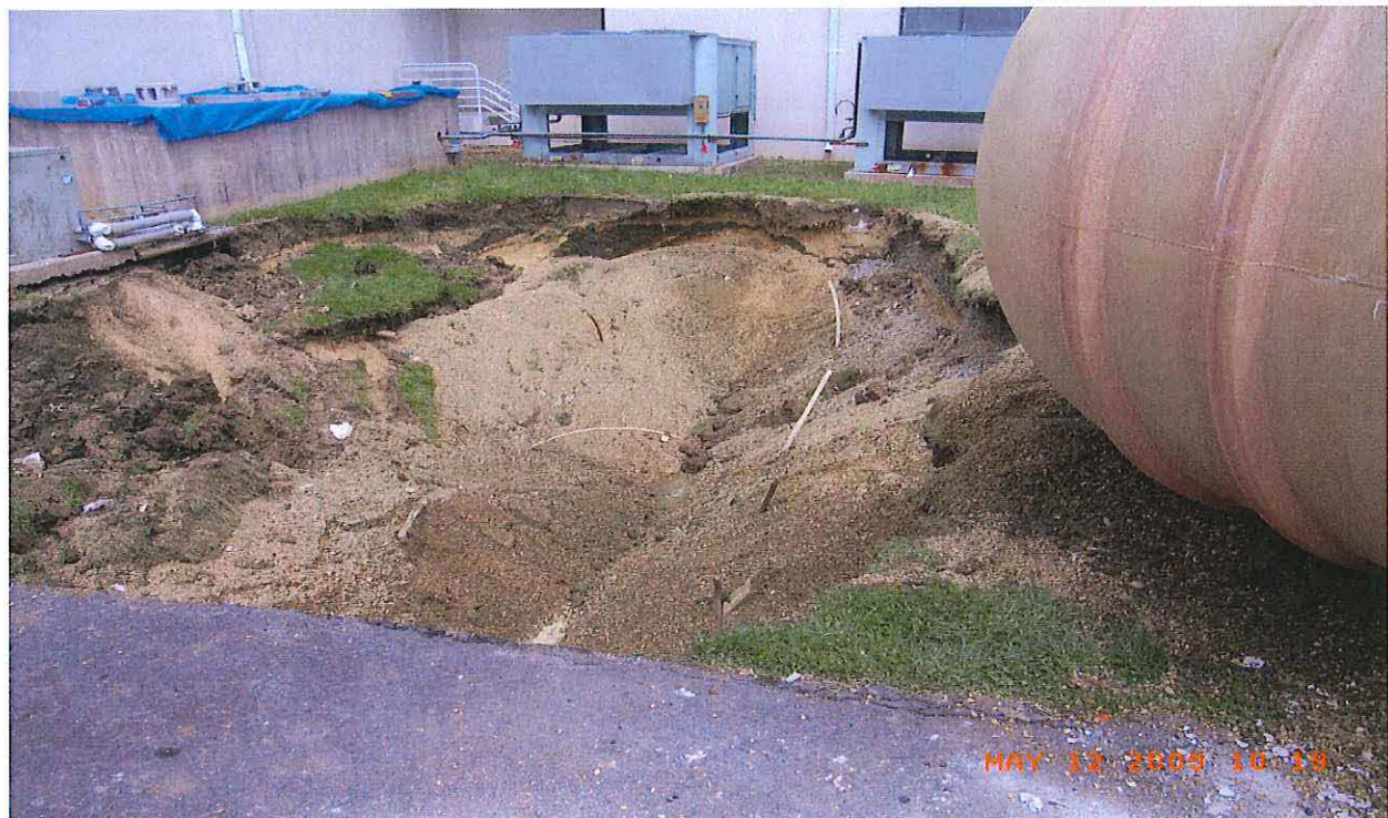
Tank excavation w/tank out of ground
