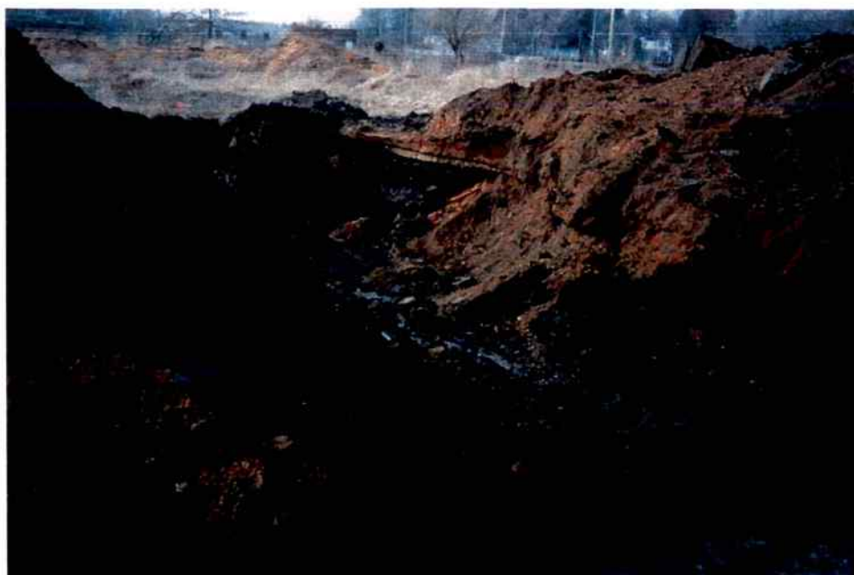
REMEDiation FROM BENEATH FORMER PIPING NEAR FORMER AST #1
