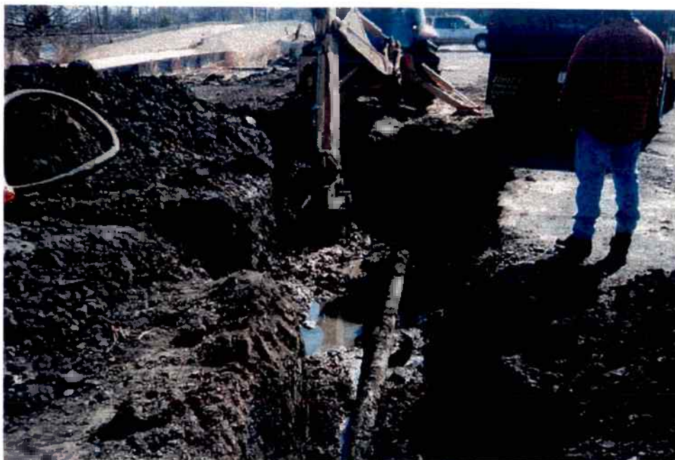
REMEDICATION OF FORMER TRUCK LOADING AREA
