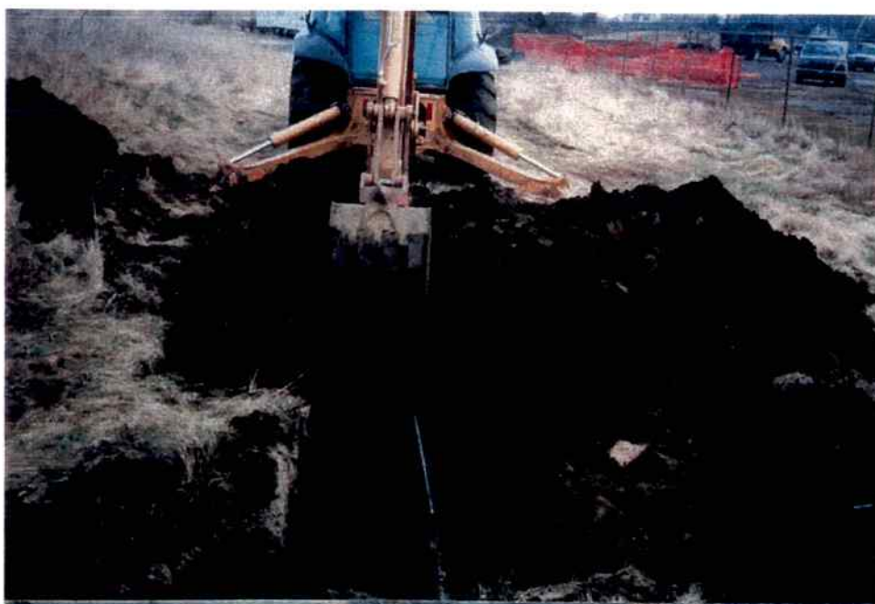
EXCAVATION AND REMOVAL OF FORMER PIPING RUN
