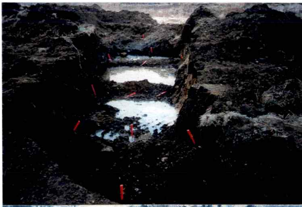
REMEDiation FROM BENEATH FORMER PIPING NEAR FORMER AST #2
