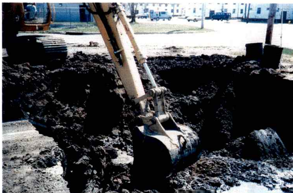
REMEDATION OF FORMER TRUCK UNLOADING AREA
