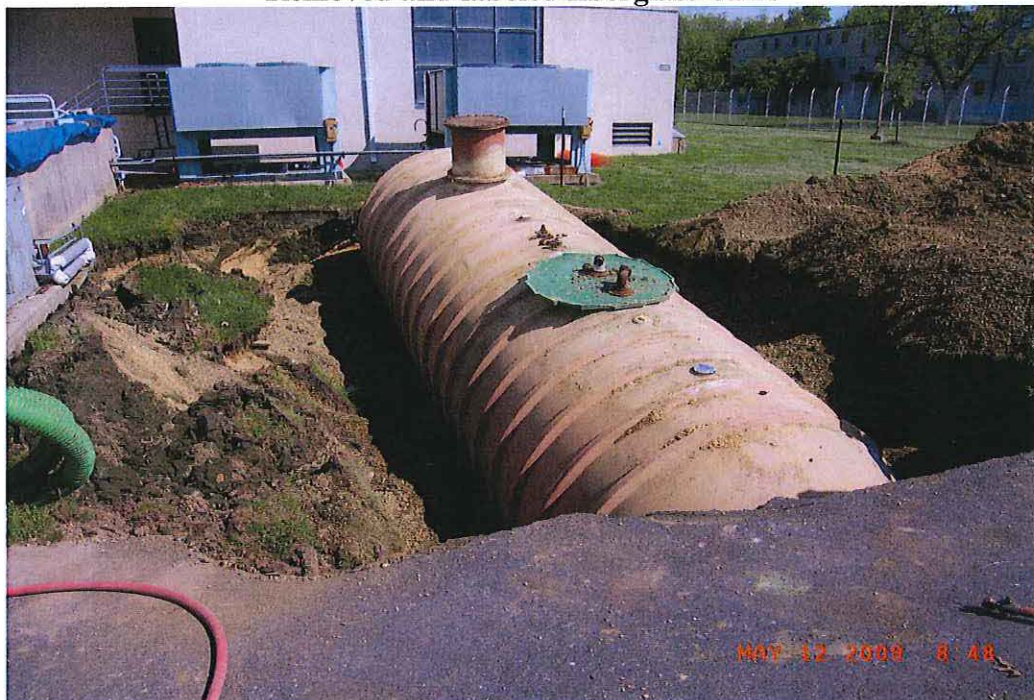
Fiberglass UST being removed from excavation
