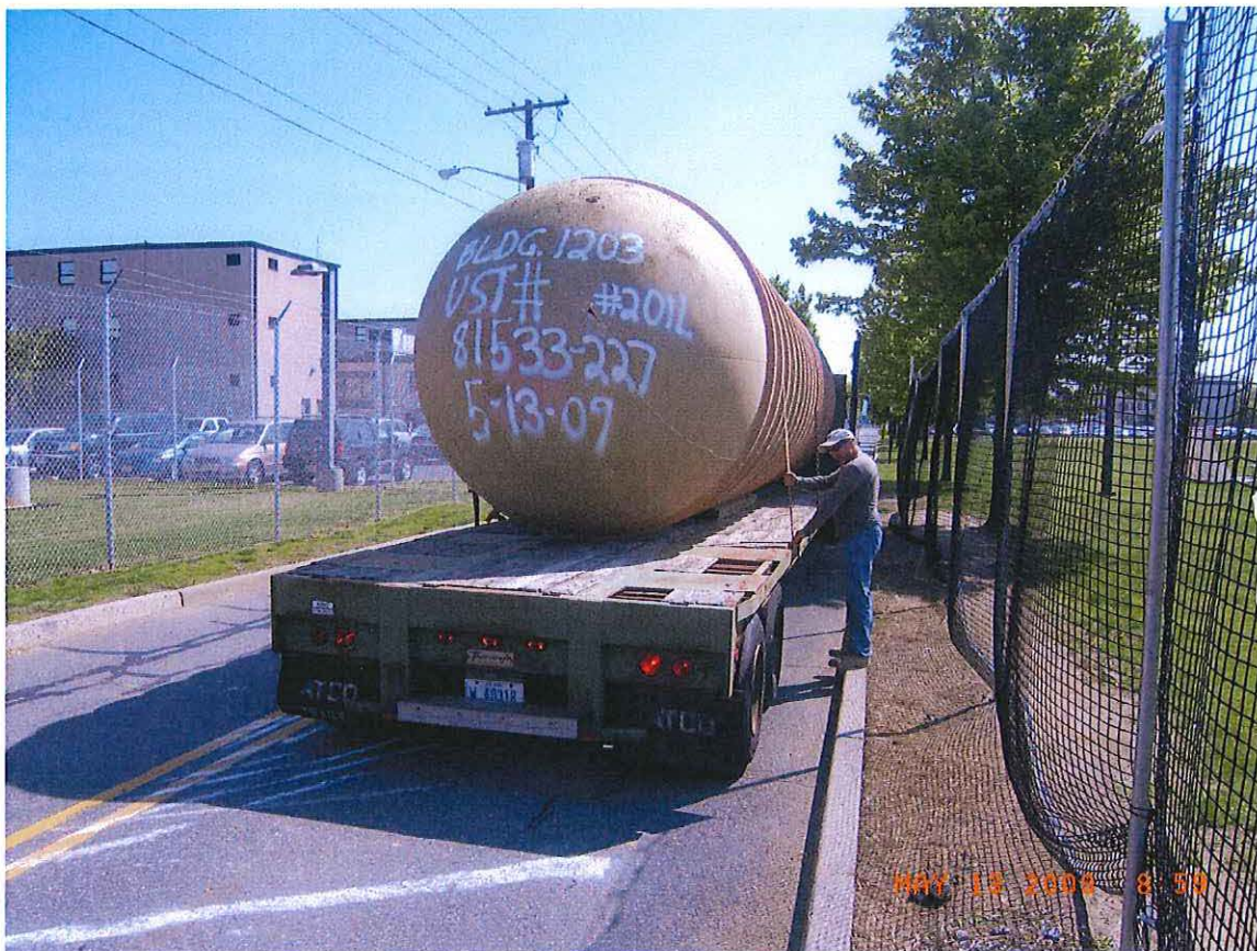
Removed and labeled fiberglass USTs
