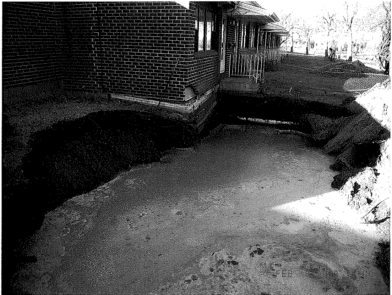
Groundwater in the excavation after the UST has been removed, note remote fill line in rear right of photograph
