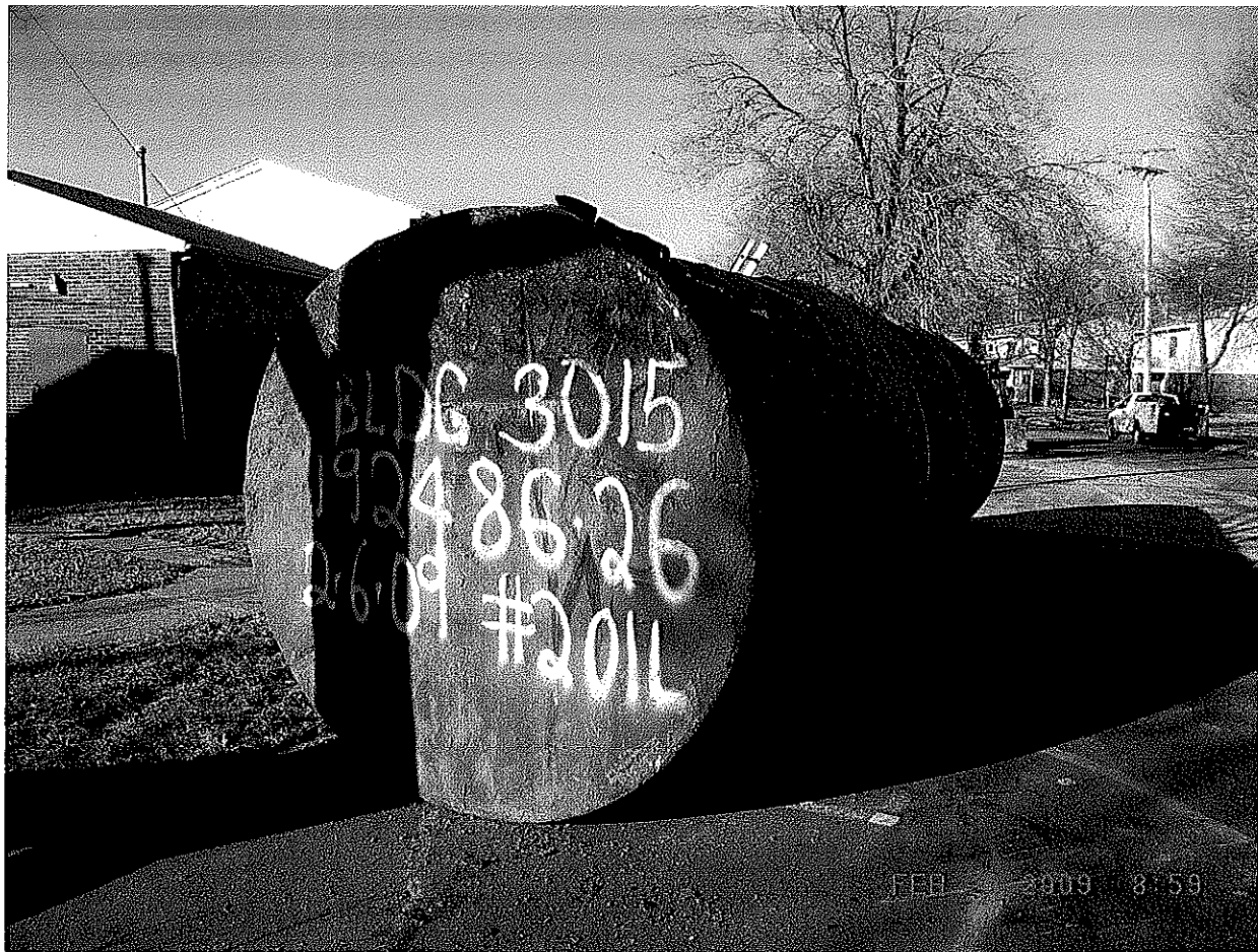
Removed and labeled steel USTs
