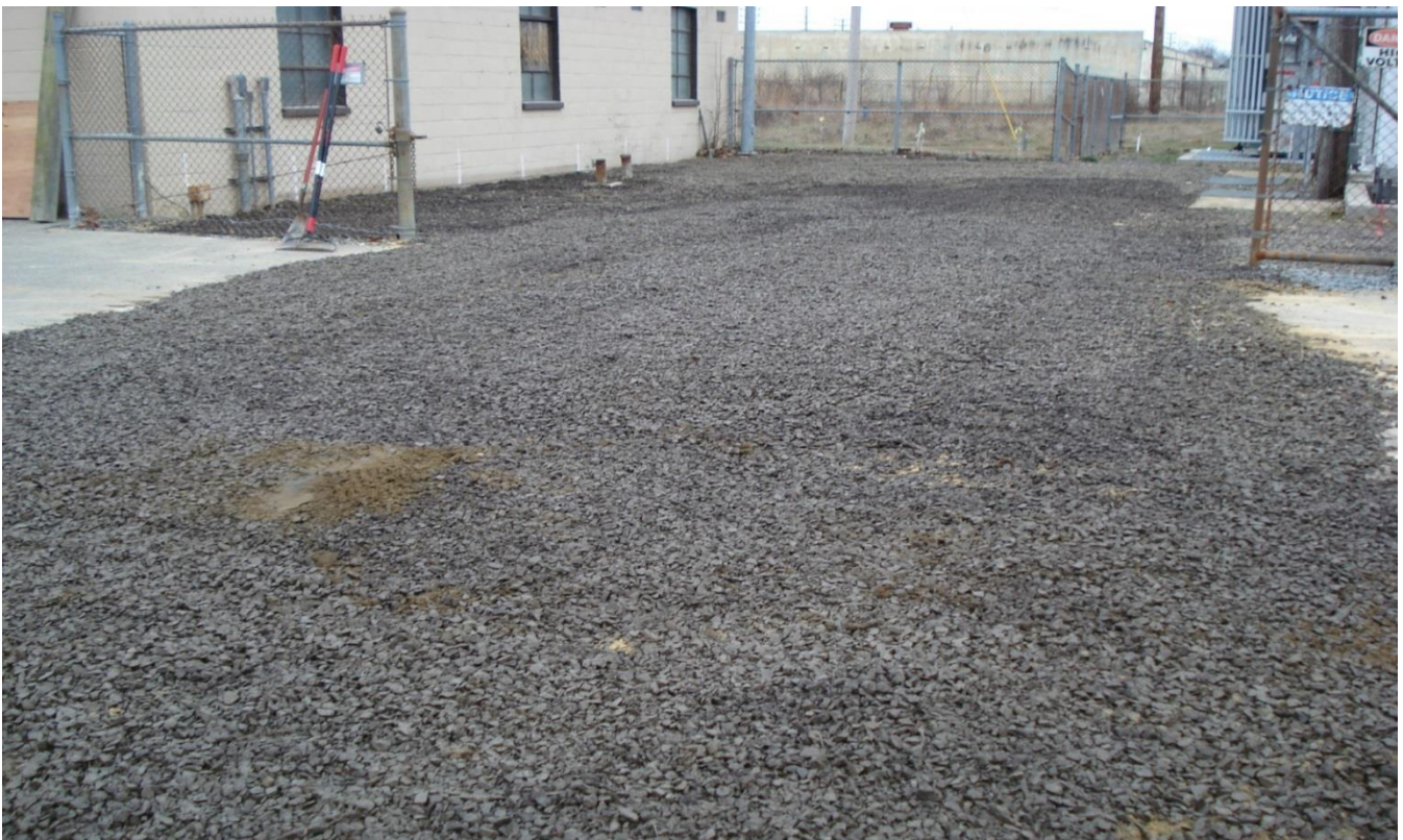
Photograph 10. Building 978, excavation after backfill completed, view east, 8 January 2016.
