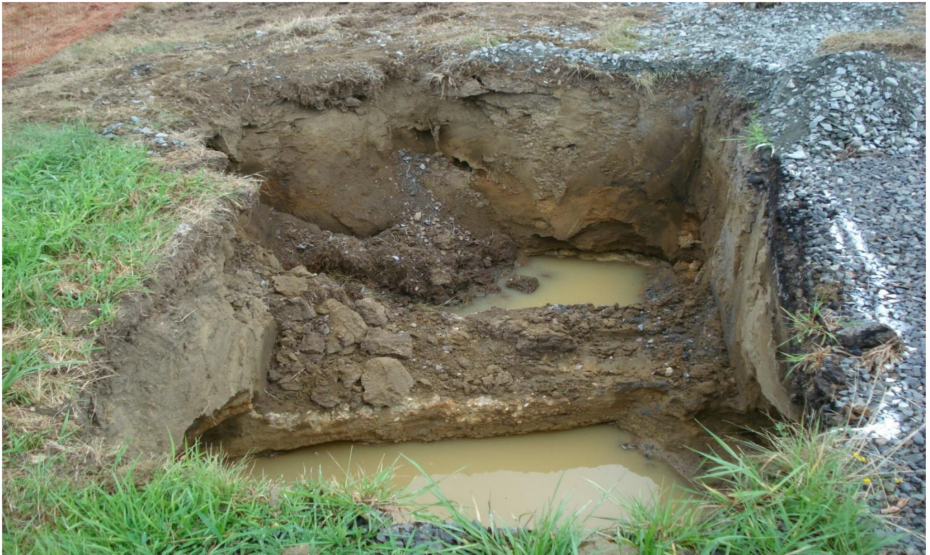
Photograph 13. Building 978, excavation at S038, view north, 25 July 2016.
