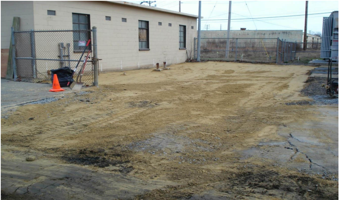
Photograph 9. Building 978, compacted soil backfill, view east, 8 January 2016.
