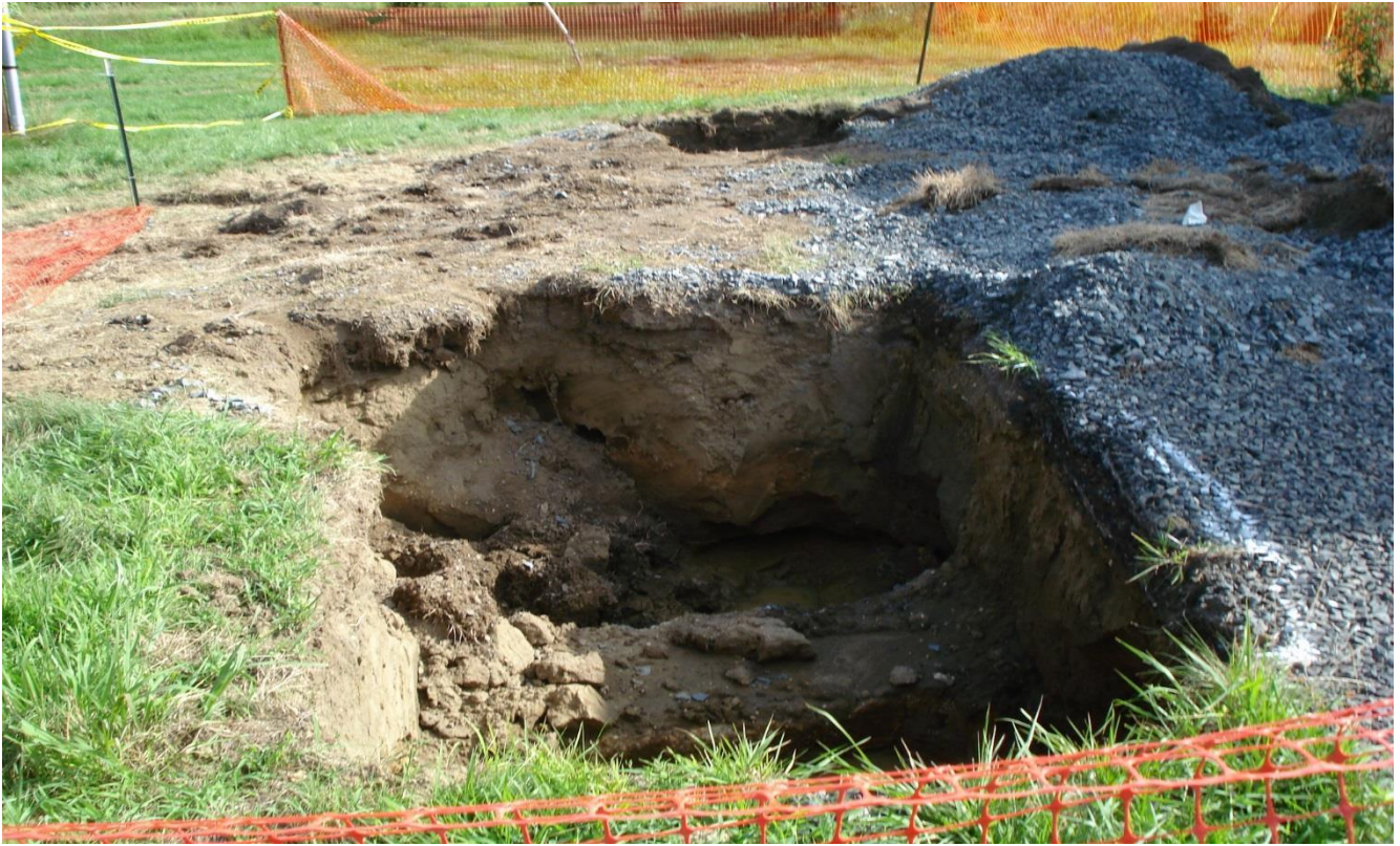
Photograph 15. Building 978, excavation at S038, view north, 27 July 2016.
