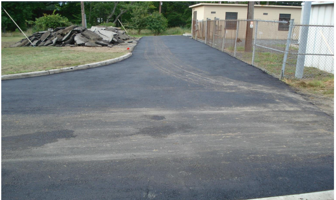
Photograph 29. Building 978, driveway paving completed, view north, 25 August 2016.
