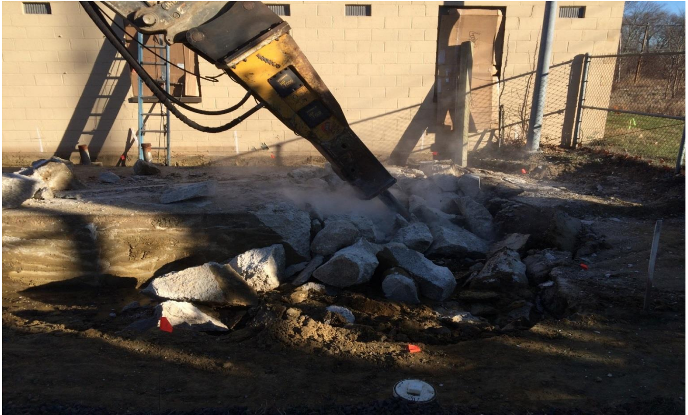
Photograph 5. Building 978, concrete pad removal, view north, 6 January 2016.
