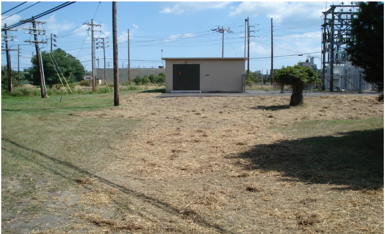
Photograph 31. Building 978, excavations at S038 and S048 seeded, view east, 26 August 2016.
