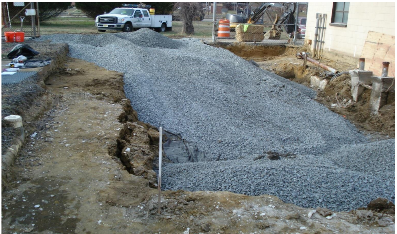
Photograph 8. Building 978, gravel backfill, view west, 7 January 2016.
