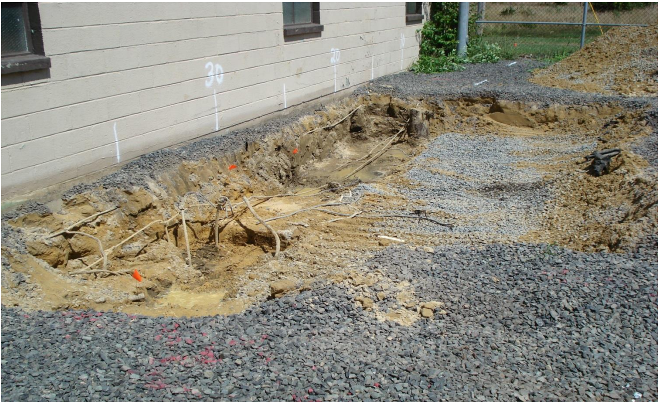
Photograph 18. Building 978, Area 1 excavation and Area 2 fill removed prior to excavation to 5 feet below ground surface, view east, 19 July 2016.
