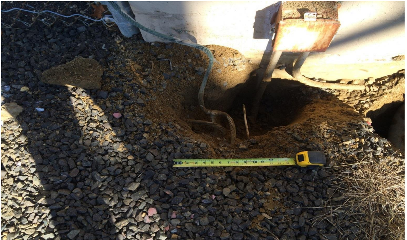
Photograph 2. Building 978, utility clearance prior to excavating, view north, 4 January 2016.
