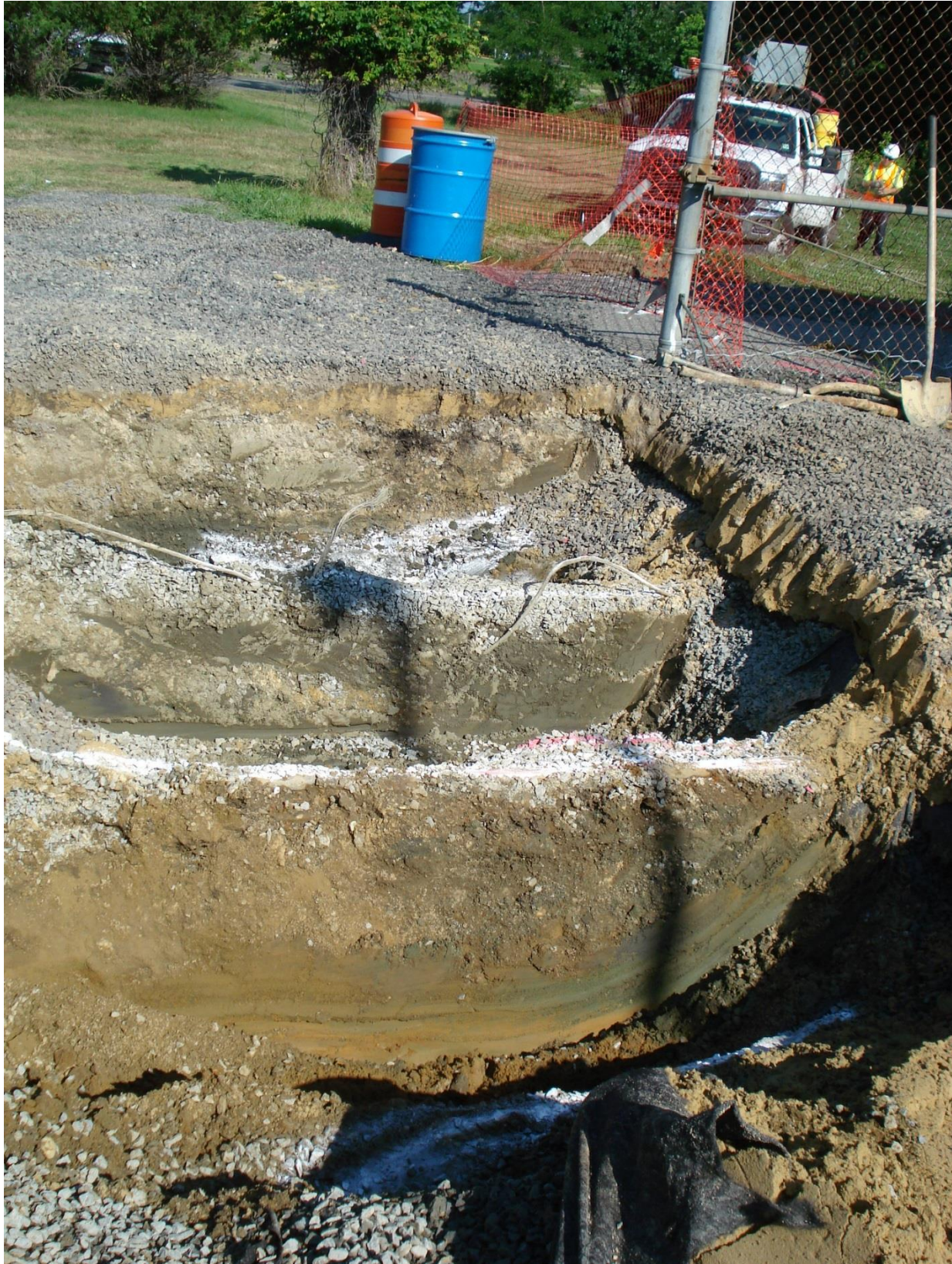
Photograph 25. Building 978, excavation between electrical lines at Area 3, view west, 21 July 2016.
