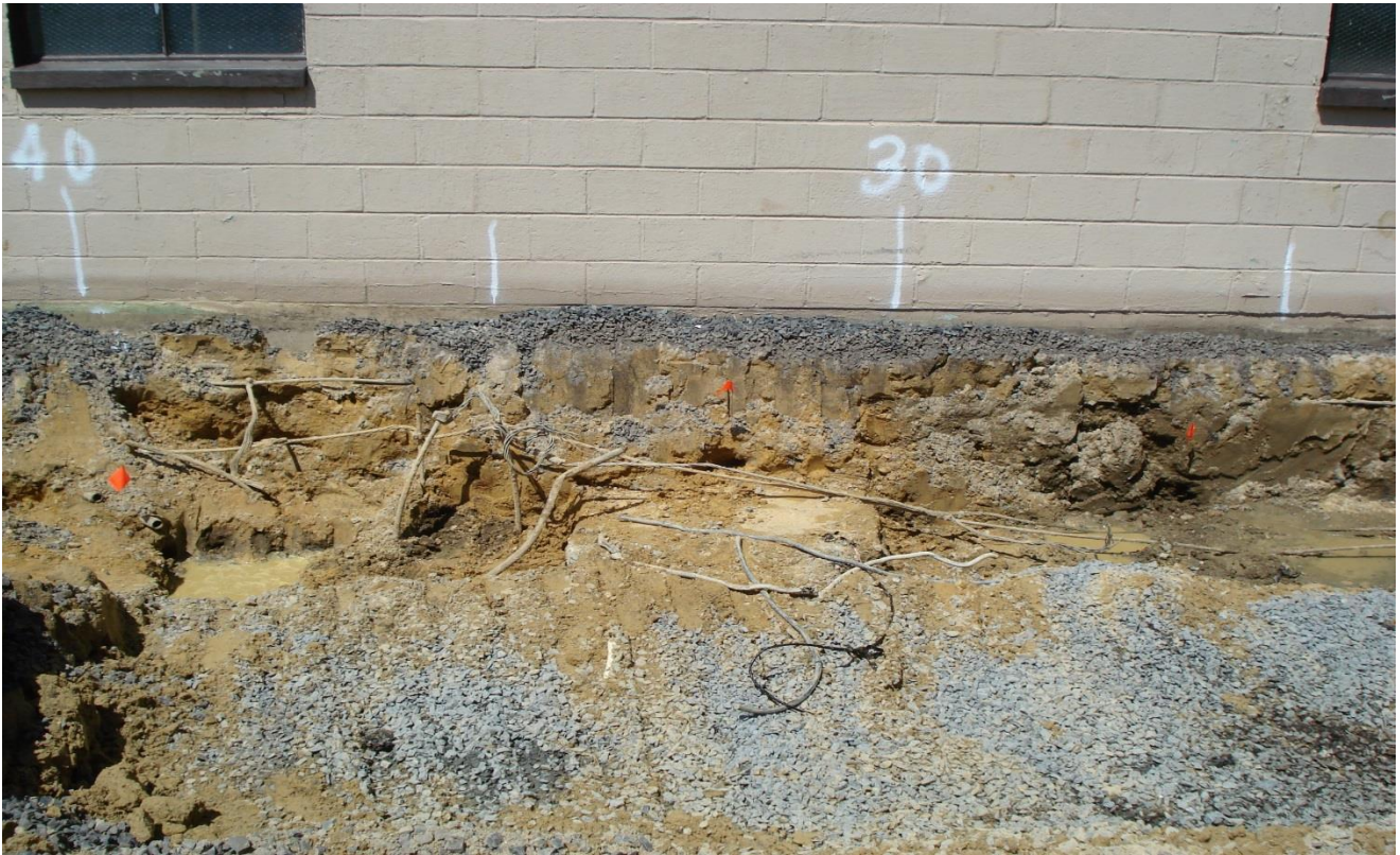
Photograph 17. Building 978, electrical and ground wires at excavation along south side of building at Area 1 excavation, view north, 19 July 2016.
