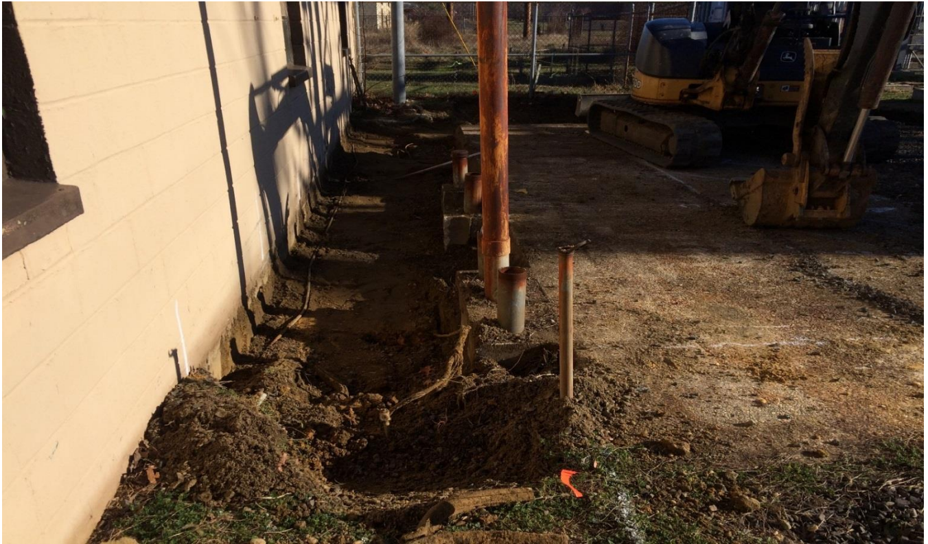
Photograph 3. Building 978, soil excavation between Building 978 and concrete pad, view east 4 January 2016.
