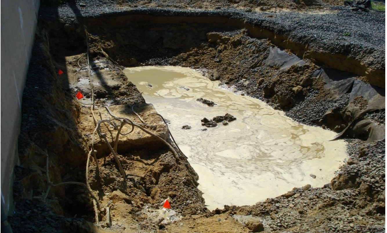
Photograph 21. Building 978, Area 1 and Area 2 excavations, view east, 20 July 2016.
