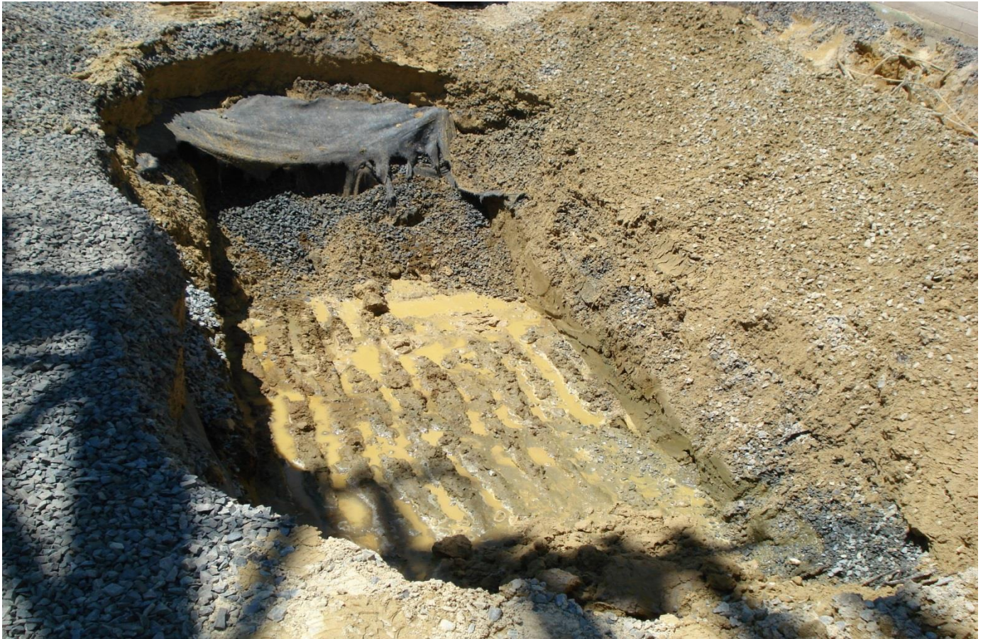
Photograph 23. Building 978, Area 4 excavated to 4 feet below ground surface, view west, 20 July 2016.
