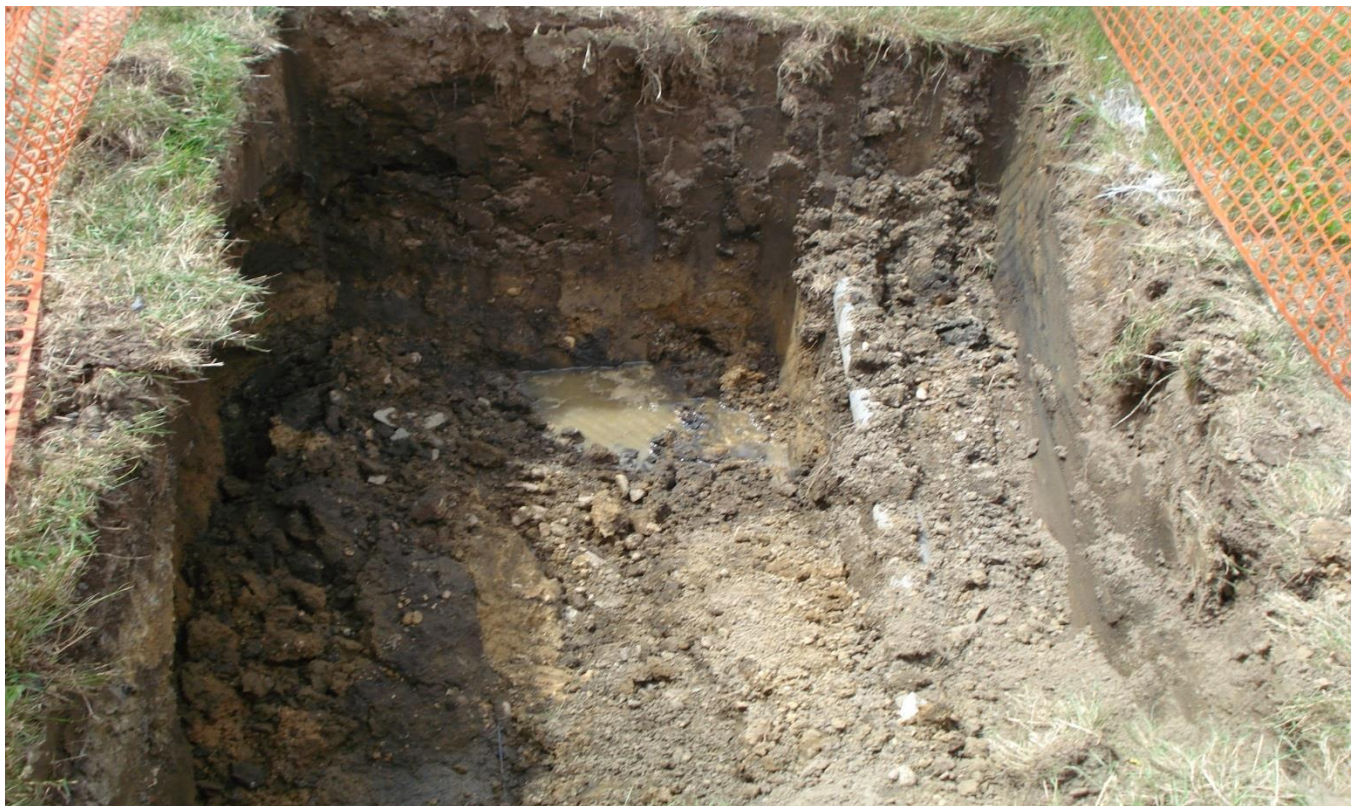
Photograph 12. Building 978, excavation at S048, view west, 18 July 2016.
