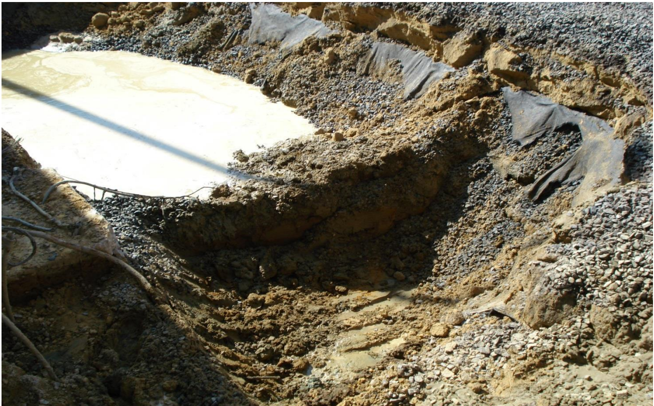
Photograph 20. Building 978, Area 2 excavation, view east, 20 July 2016.
