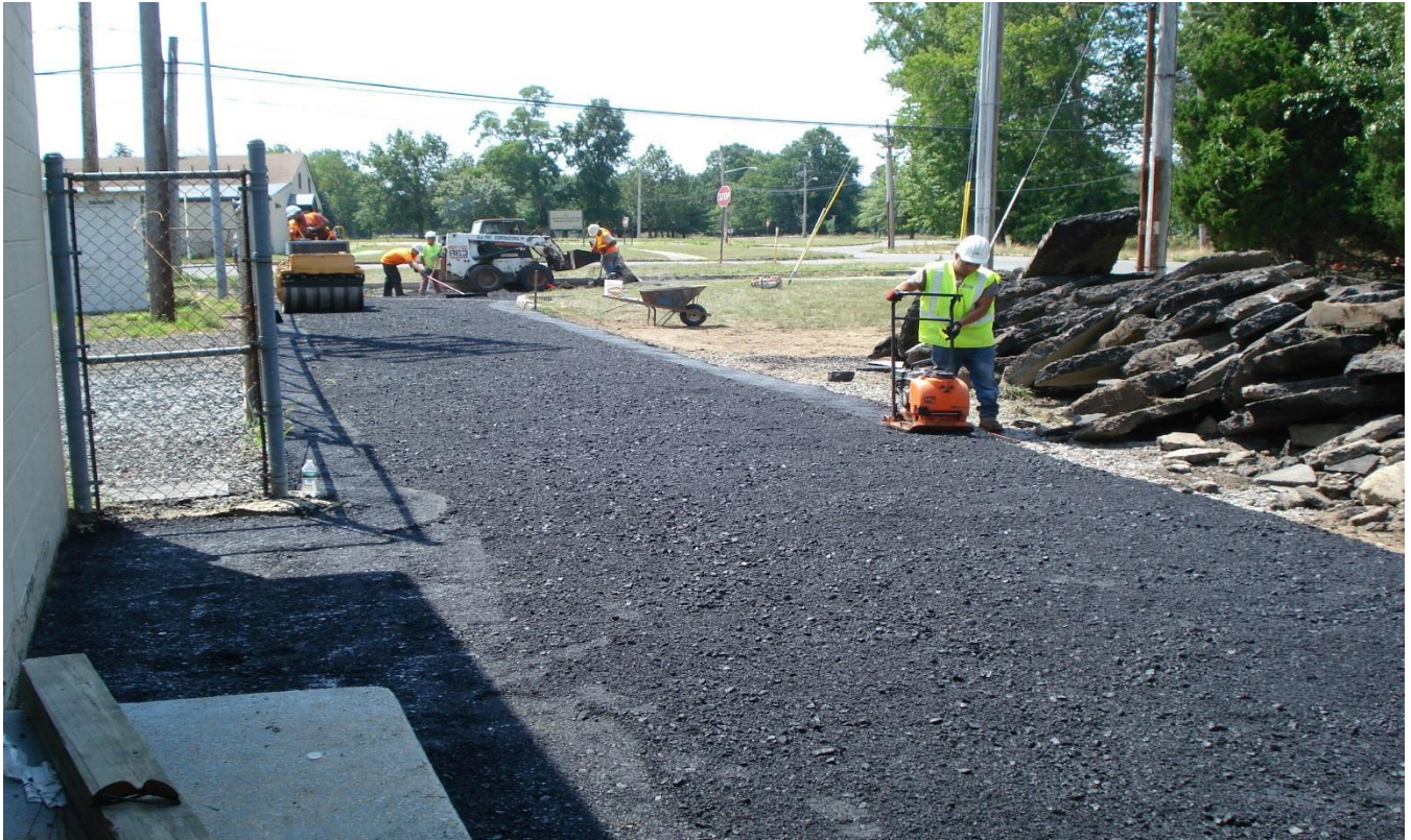
Photograph 28. Building 978, driveway paving, view south, 25 August 2016.
