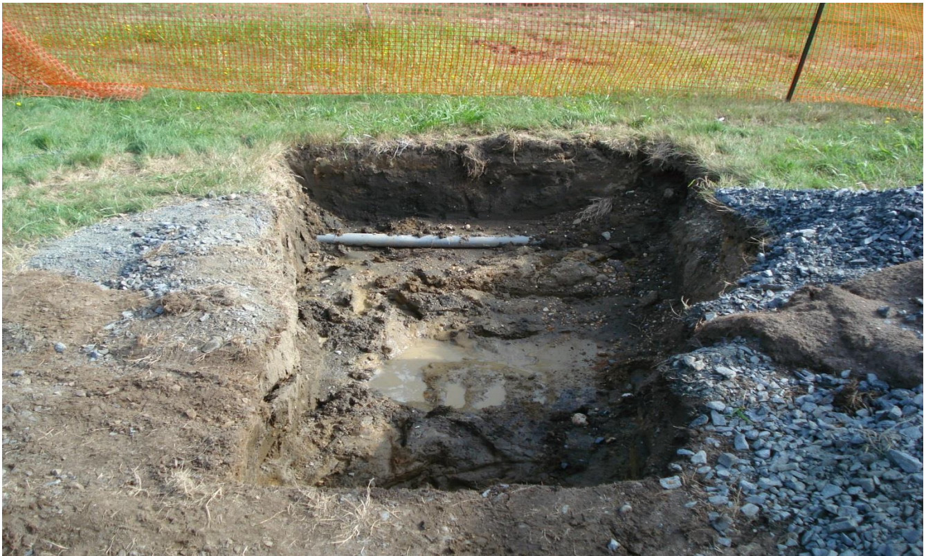
Photograph 16. Building 978, excavation at S048, view north, 27 July 2016.
