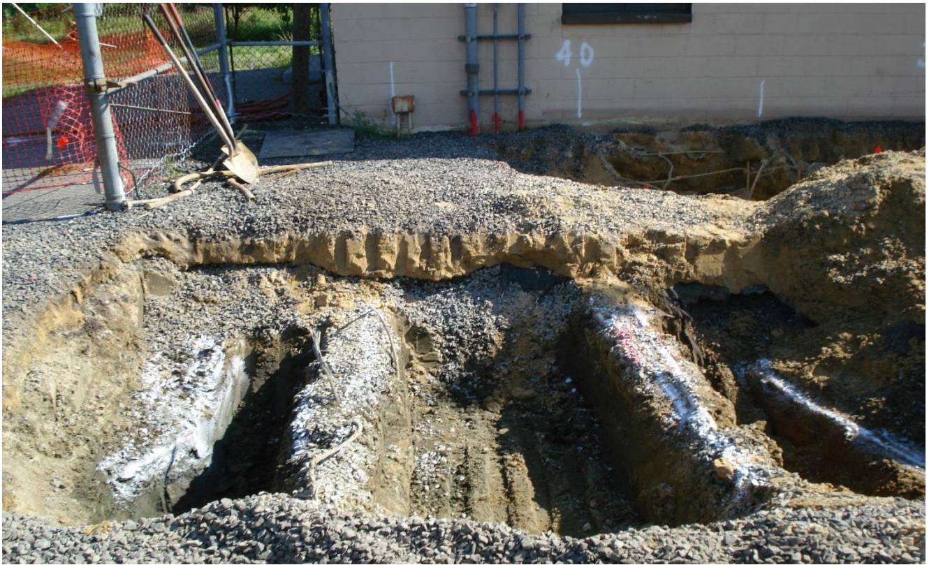
Photograph 26. Building 978, excavation between electrical lines at Area 3, view north, 21 July 2016.
