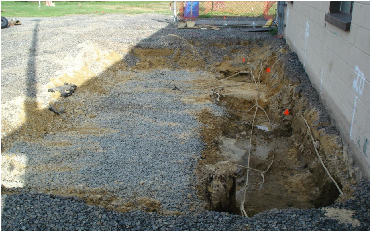
Photograph 19. Building 978, Area 1 excavation completed and fill removed at Area 2, view west, 20 July 2016.
