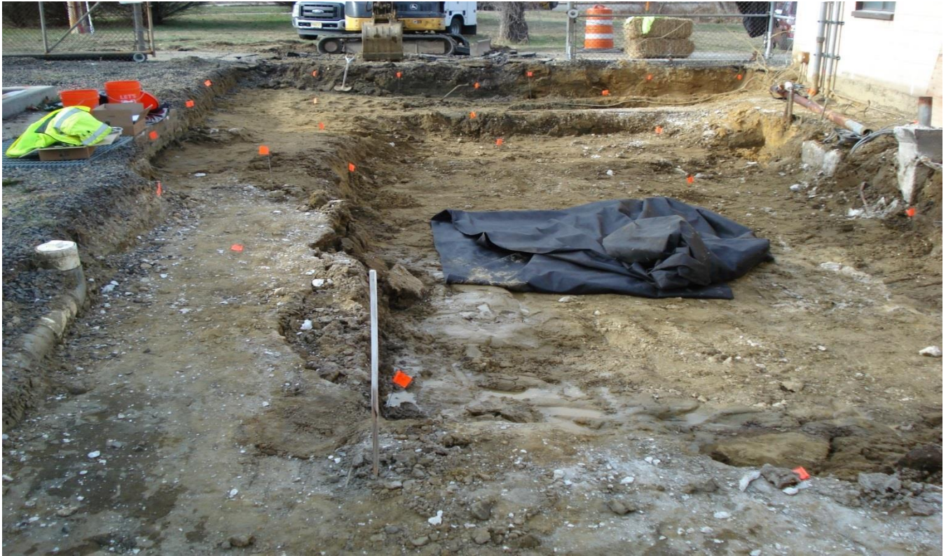
Photograph 7. Building 978, post excavation, view west, 7 January 2016.
