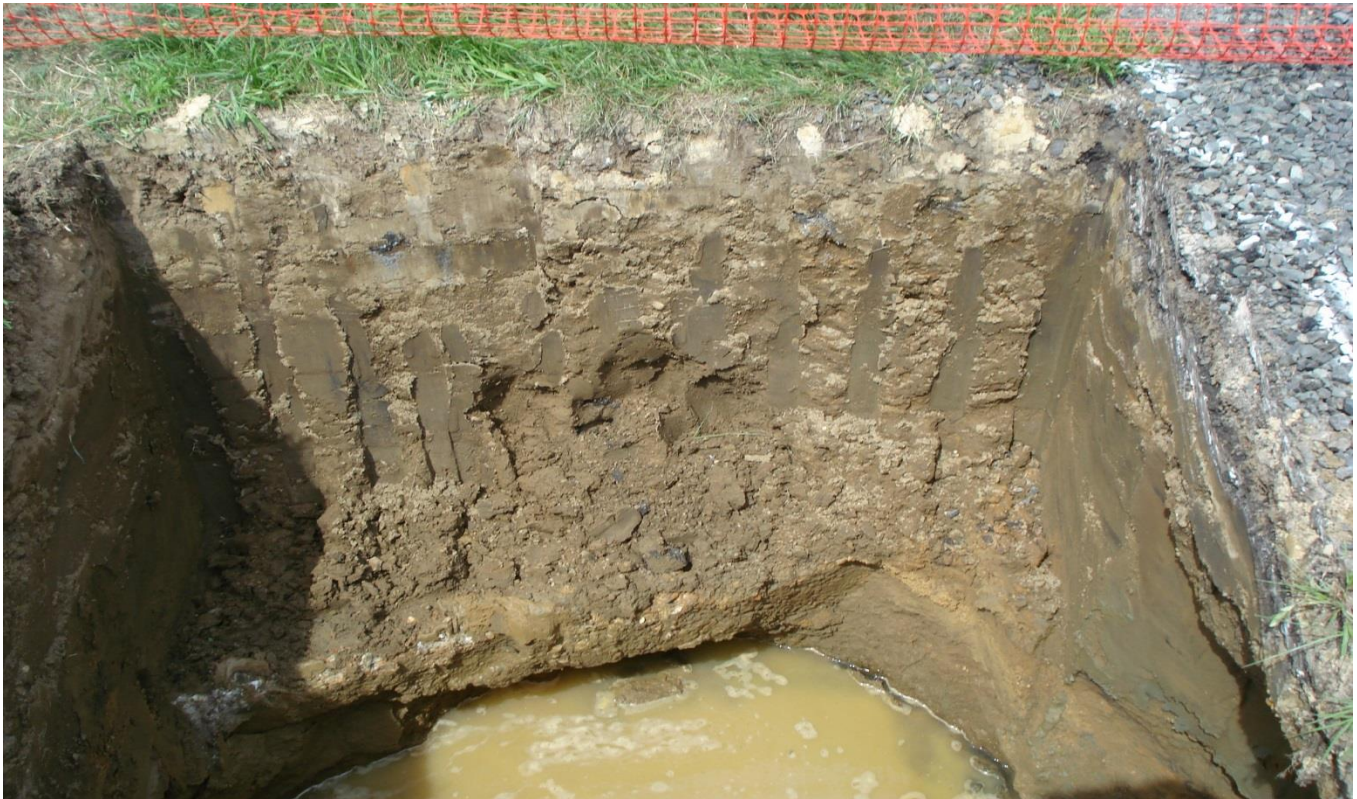
Photograph 11. Building 978, north wall of excavation at S038 to five feet, view north, 18 July 2016.
