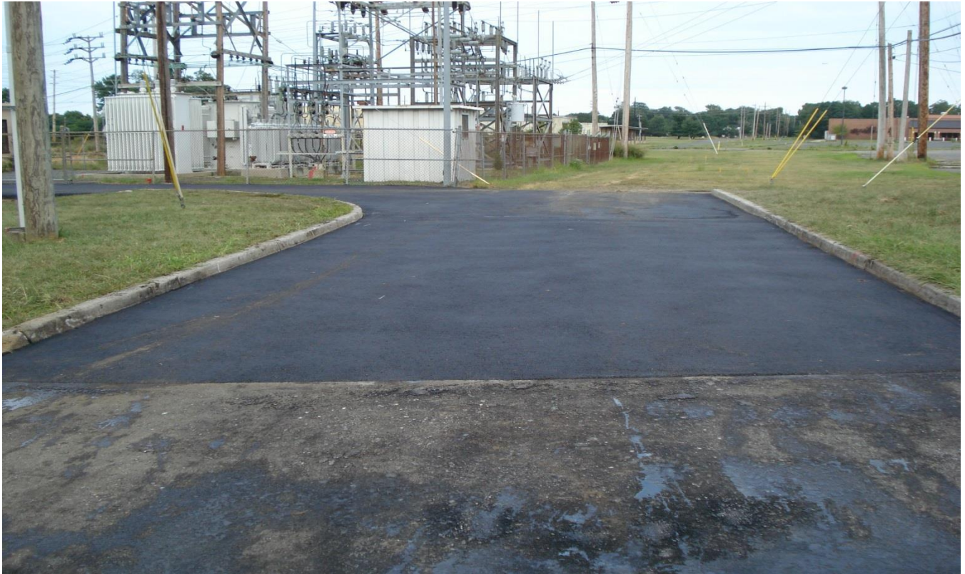
Photograph 30. Building 978, driveway paving completed, view east, 25 August 2016.
