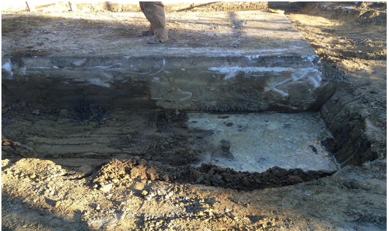
Photograph 4. Building 978, concrete pad and water in excavation, view north 5 January 2016.
