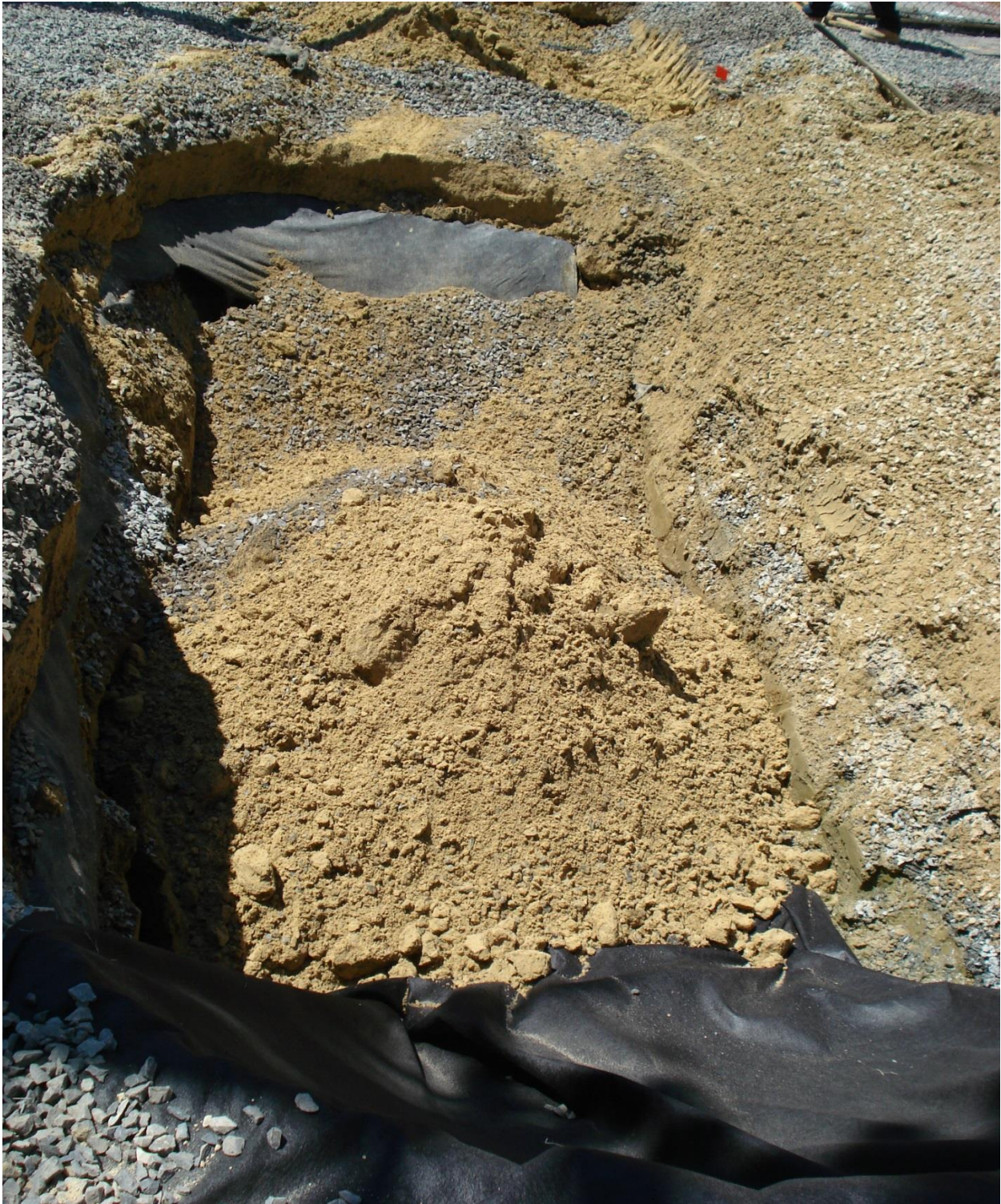
Photograph 24. Building 978, backfilling at Area 4 excavation, view west, 20 July 2016.
