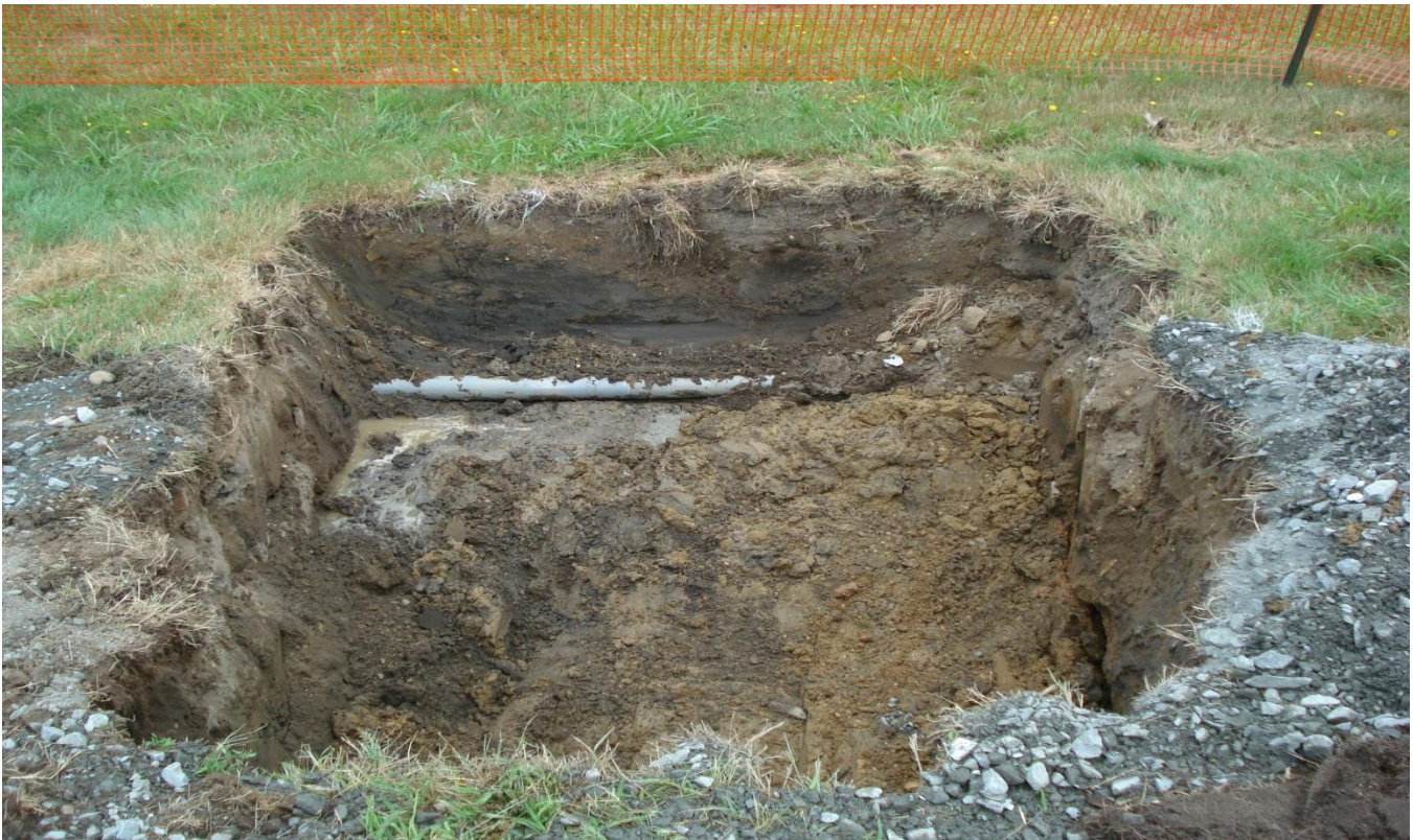
Photograph 14. Building 978, excavation at S048, view north, 25 July 2016.
