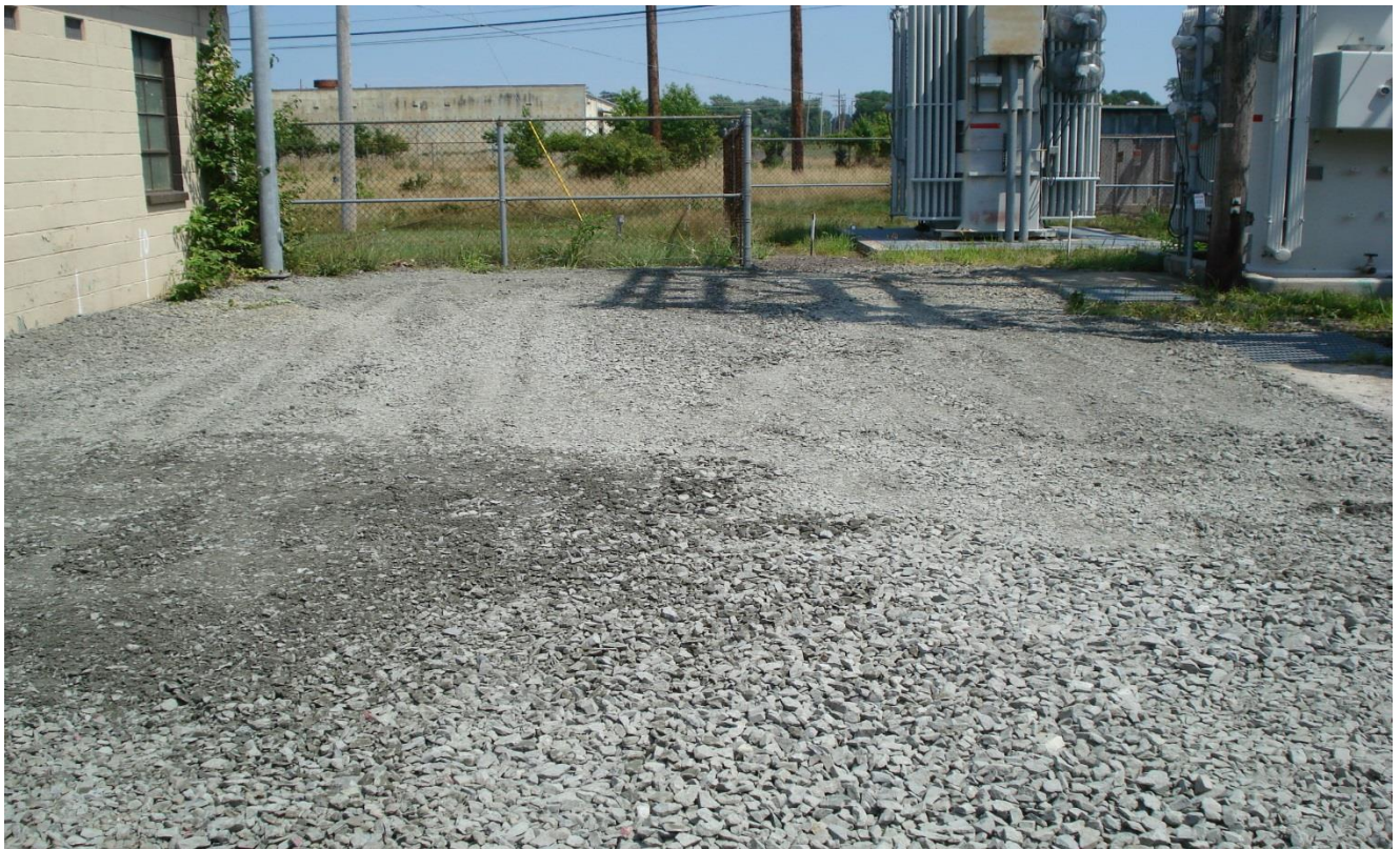
Photograph 27. Building 978, backfilled excavations, view east, 25 July 2016.
