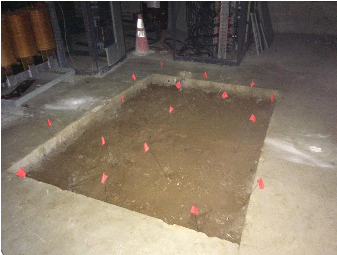
Photograph 3. Building 1002, PCB soil and concrete sample locations, view north, 18 December 2015.
