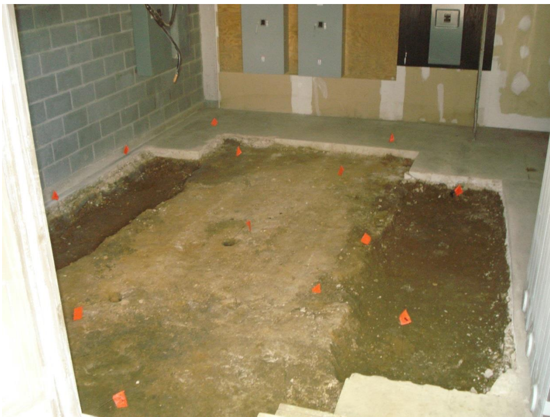
Photograph 2. Building 1208, PCB soil sample locations, view north, 2 August 2016.
