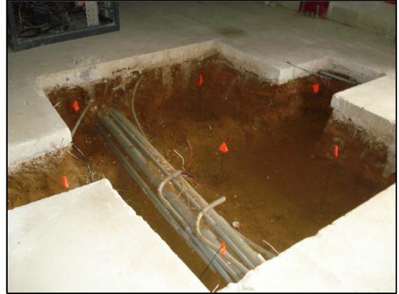
Figure 3 - Building 1002 Excavation and PCB Soil Sample Locations, August 2016
