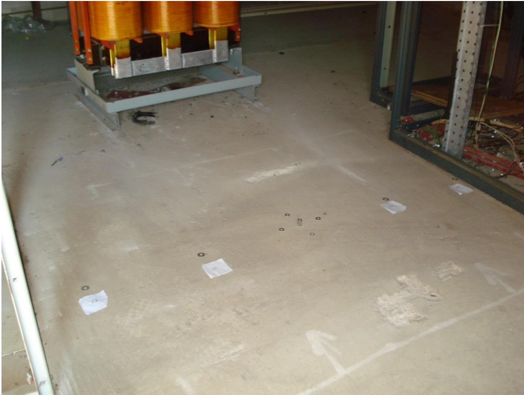
Photograph 1. Building 1002, PCB concrete sampling locations S3, S1, S2, and S4 from left to right in photo, view west, 13 October 2015.
