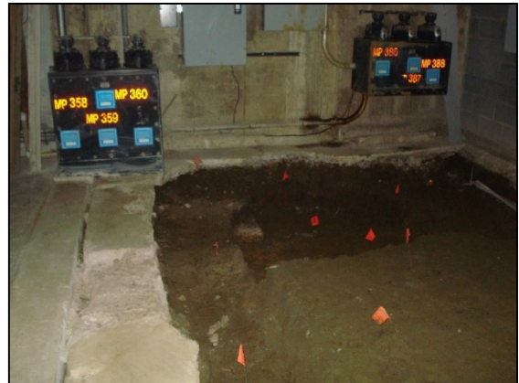
Figure 5 - Building 1209 Excavation and PCB Soil Sample Locations, August 2016
