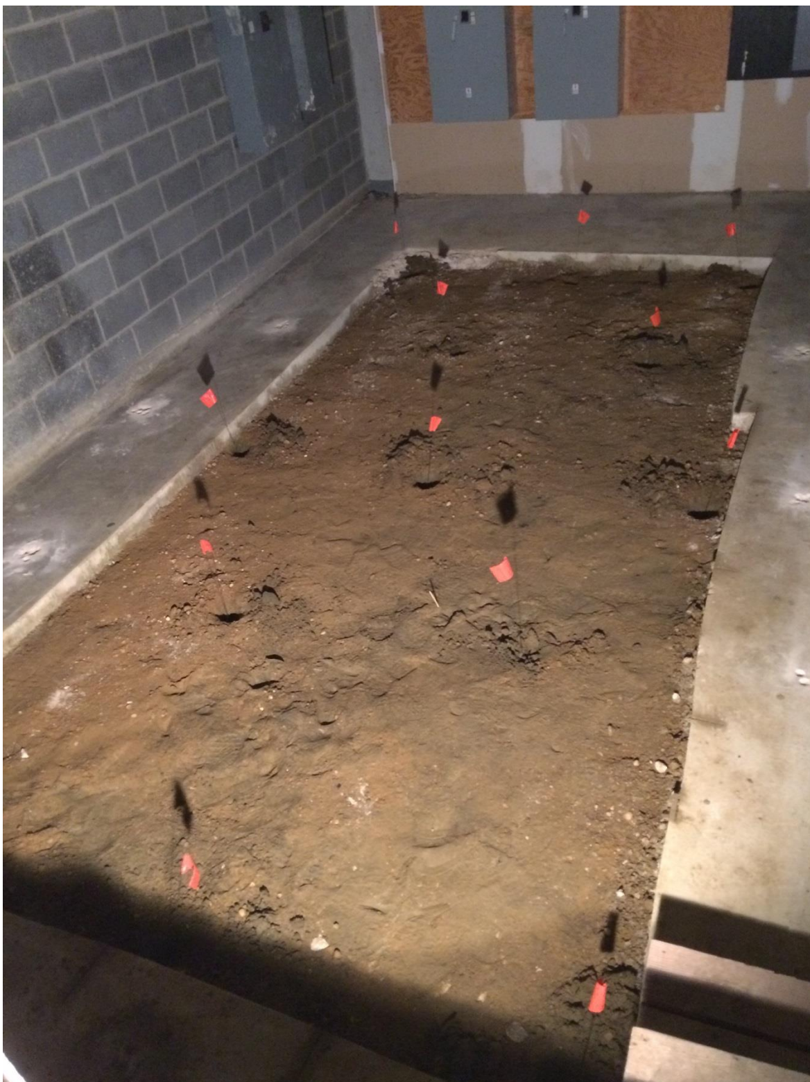
Photograph 1. Building 1208, PCB soil and concrete sample locations, view north, 18 December 2015.
