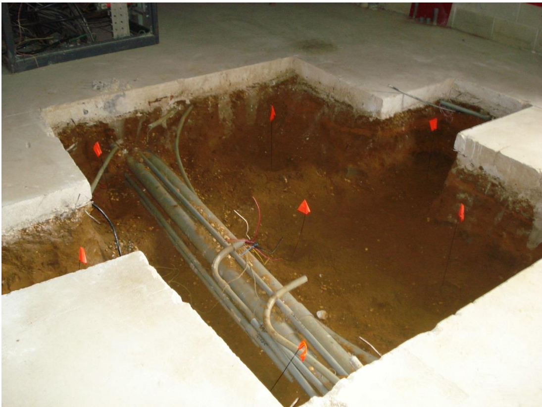
Photograph 4. Building 1002, PCB soil sample locations, view northeast, 2 August 2016.
