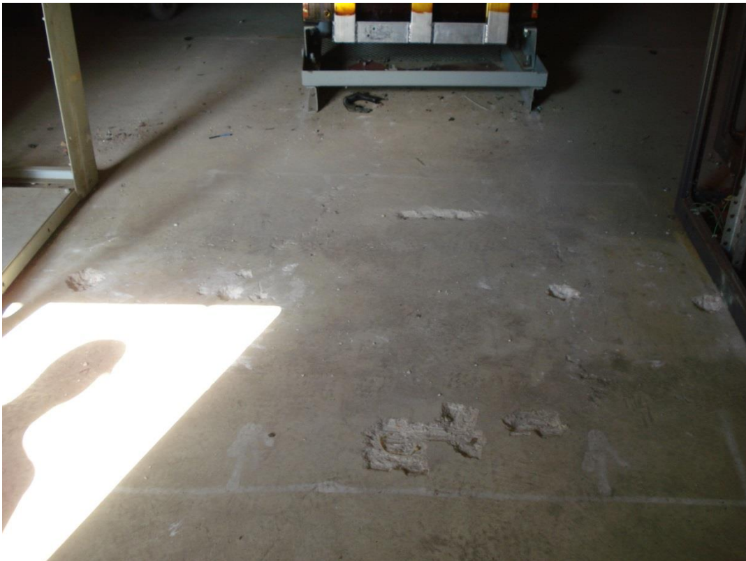
Photograph 2. Building 1002, PCB concrete sample locations, view west October 2015.
