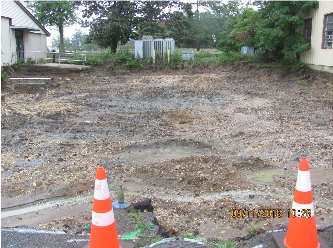
PHOTO 7 – Buildings 291/296 Excavation - Central Leg; Looking South.
