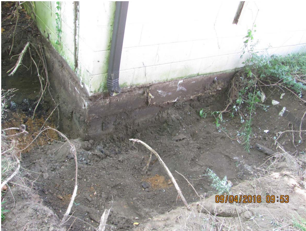
PHOTO 5 – Building 293 Excavation Cell A8; Looking South.
