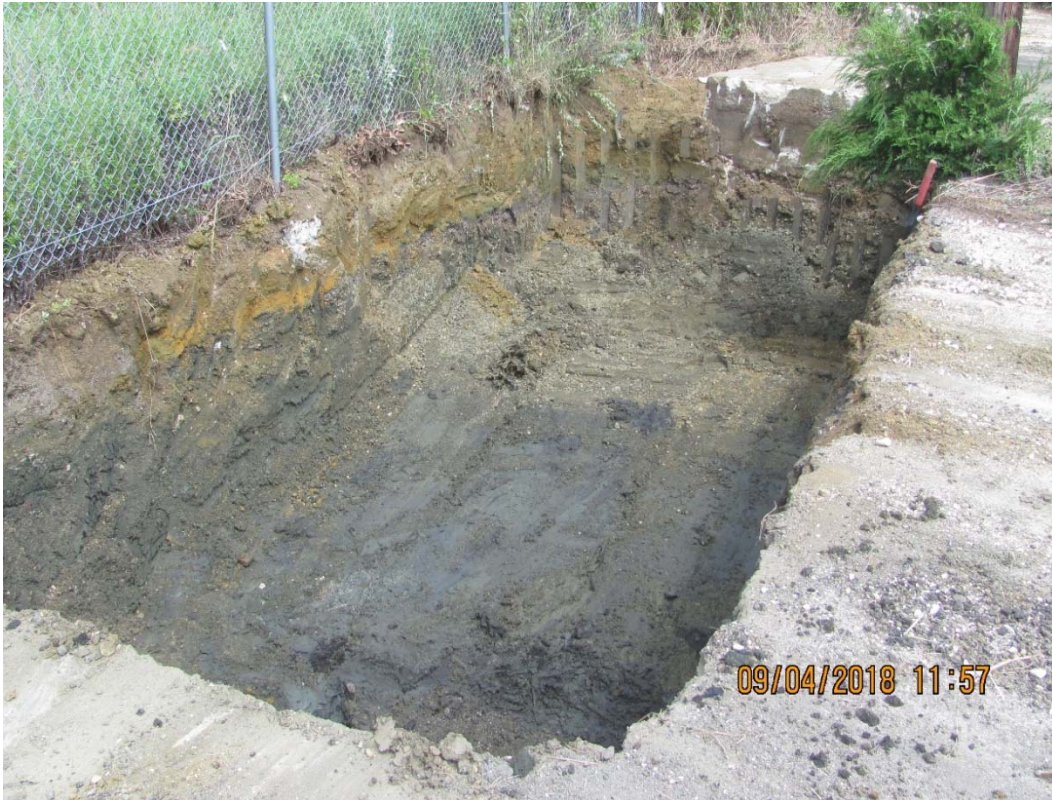
PHOTO 3 – Building 293 Excavation Cells A5, A4, and A3; Looking East.
