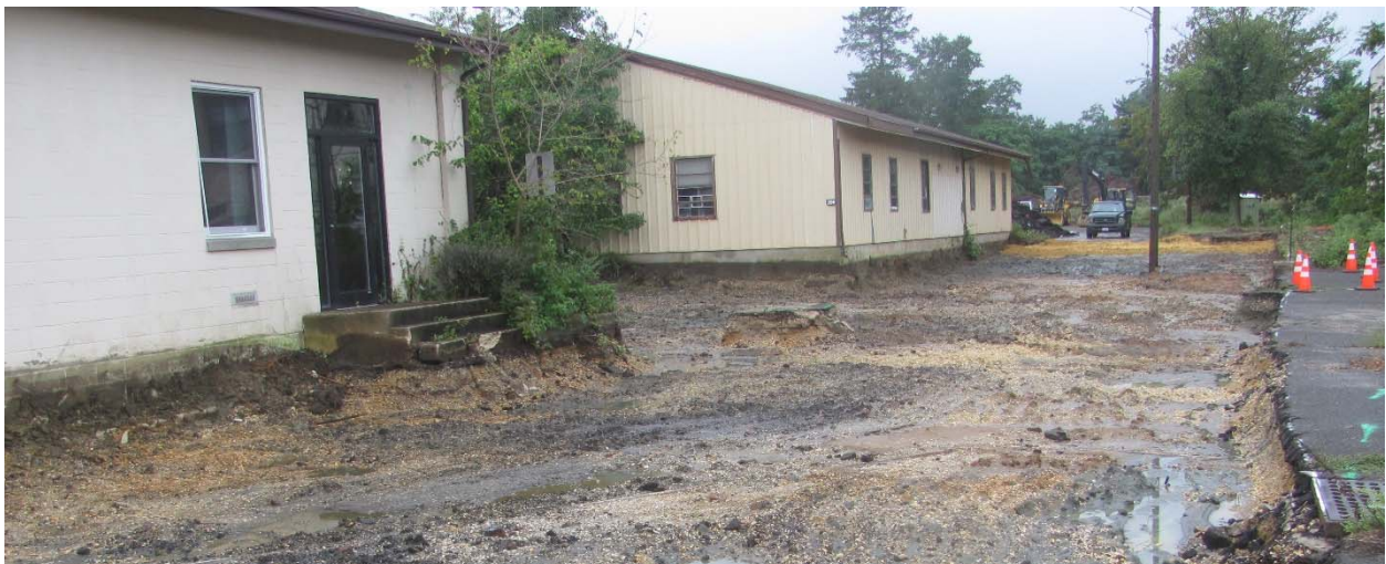
PHOTO 8 – Buildings 291/296 Excavation - Western End Leg; Looking West. Start of backfill in background.
