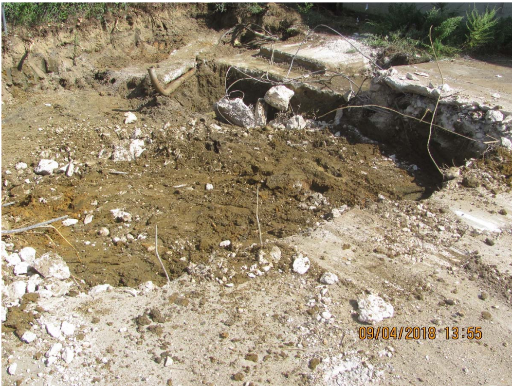
PHOTO 4 – Building 293 Excavation Cells A6 and A7; Looking East.
