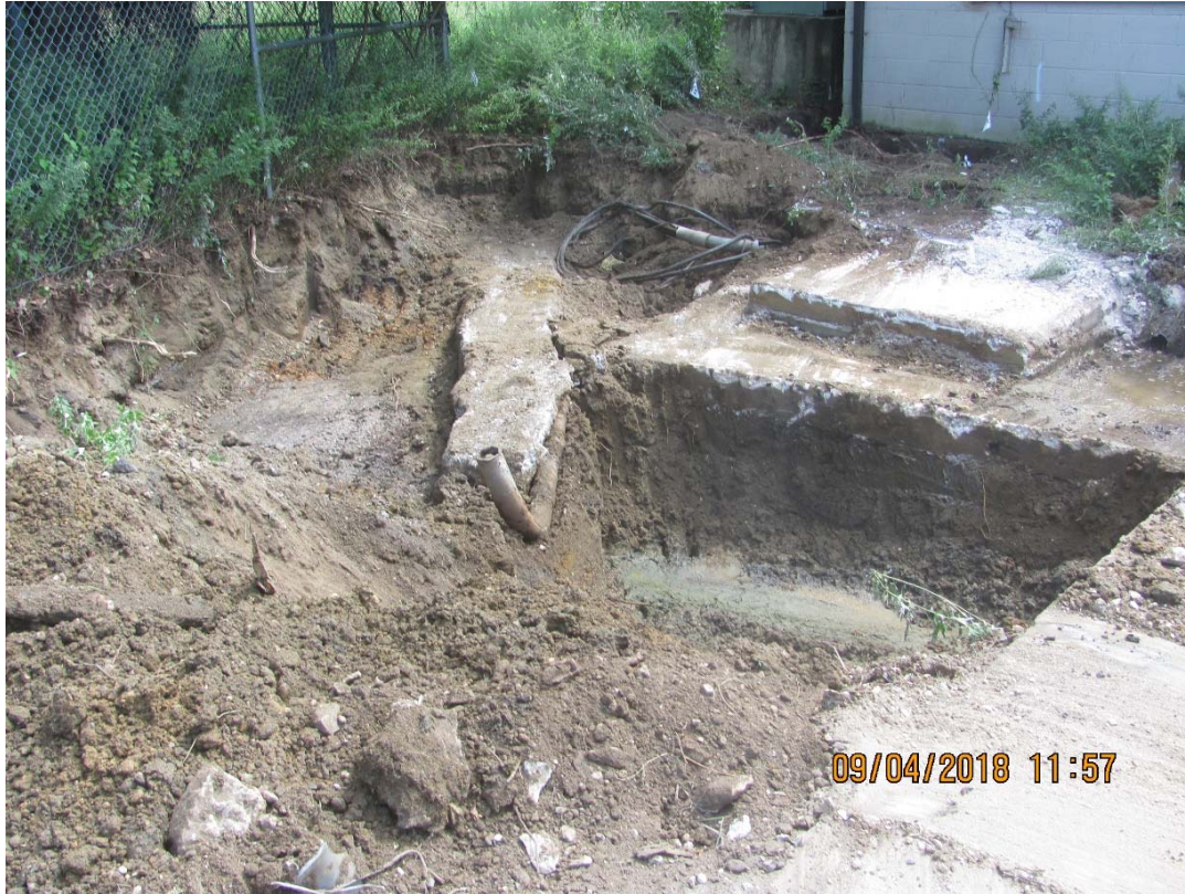
PHOTO 1 – Building 293 Excavation Cell A1; Looking East.
