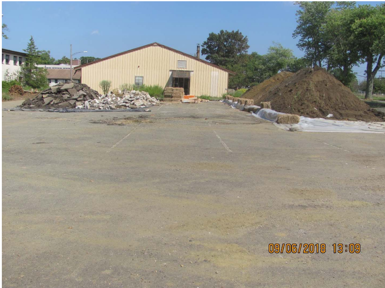
PHOTO 9 – Stockpiles area (left to right: asphalt, concrete, soil stockpiles awaiting to be covered).
