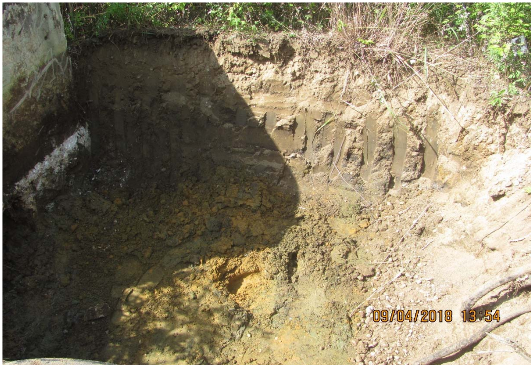
PHOTO 2 – Building 293 Excavation Cell A2; Looking West.
