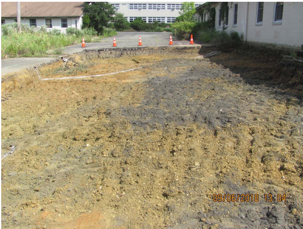
PHOTO 6 – Buildings 291/296 Excavation - Eastern Leg; Looking East.
