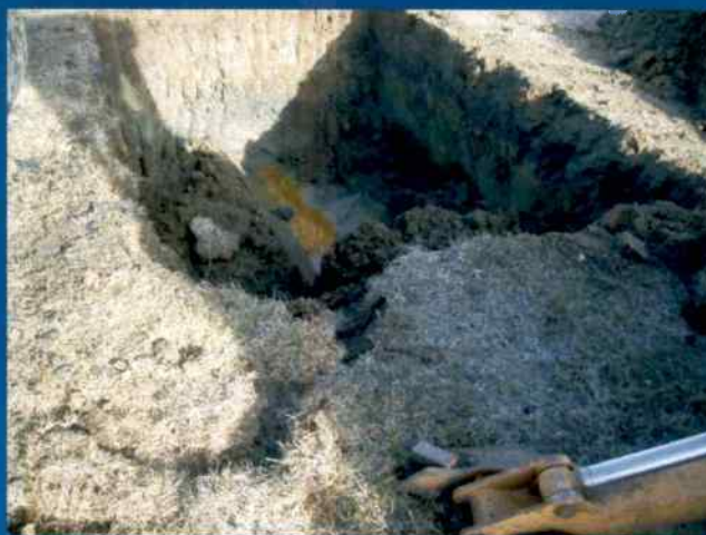
Parcel 79 Building 440 30 cubic yards of petroleum contaminated soil were excavated from the UHOT site
