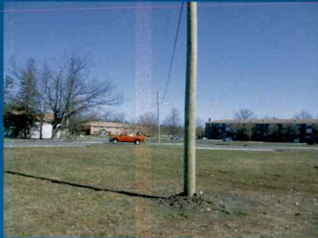
Parcel 76 New utility pole
