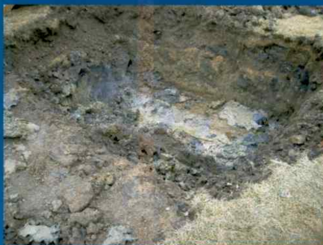
Parcel 76-6 Excavation prior to remediation
