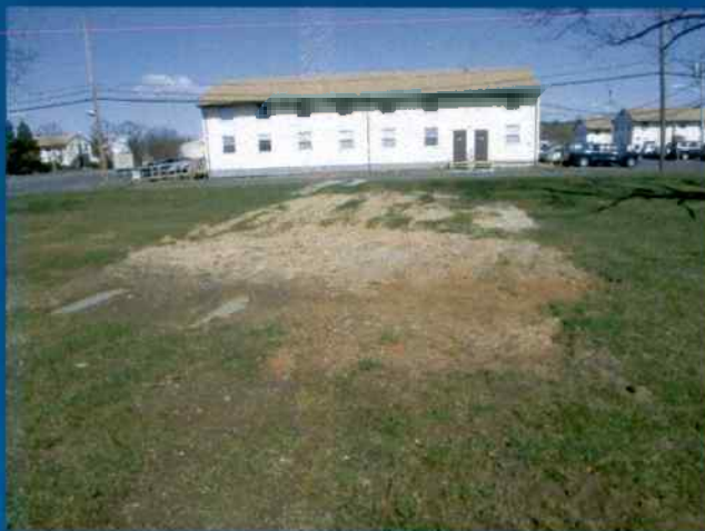
Parcel 79-12 Site after it was back filled.
