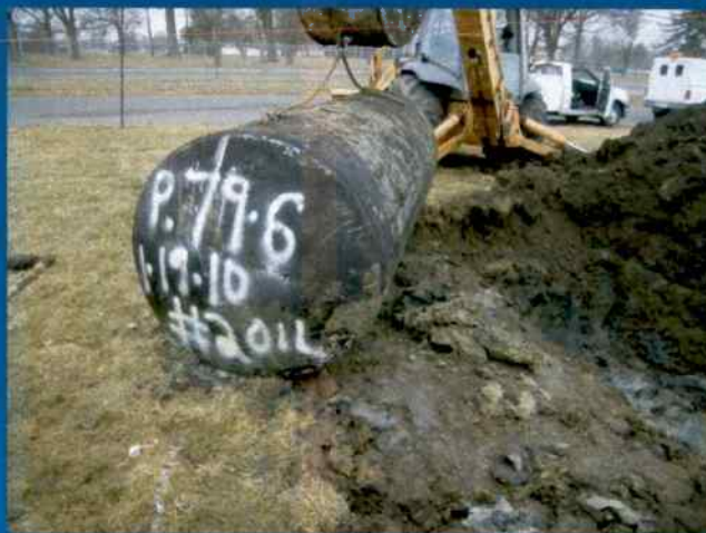
Parcel 79-6 1000-gallon UHOT Excavated 40 cubic yards of petroleum contaminated soil
