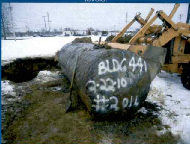
Parcel 79-18 40 cubic yards of petroleum contaminated soil were excavated from the site and transported to the soil pad adjacent to Building 490. Post excavation samples were collected and came back below regulatory levels.
