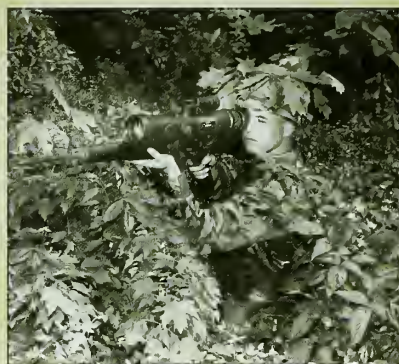
Starlight scope that intensifies moonlight, starlight, or skyglow, eliminating need for infrared light source, 21 May 1968
